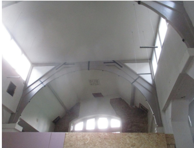
Photo 4. North wall below RF02.
