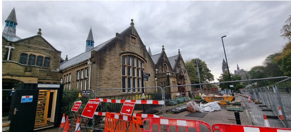
Photo 1. South elevation showing the gabled bays making up, from left to right, RF03, RF02 and RF01.
