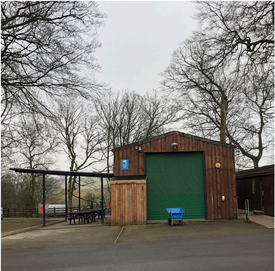
Item 1 - canopy and porch to shed
