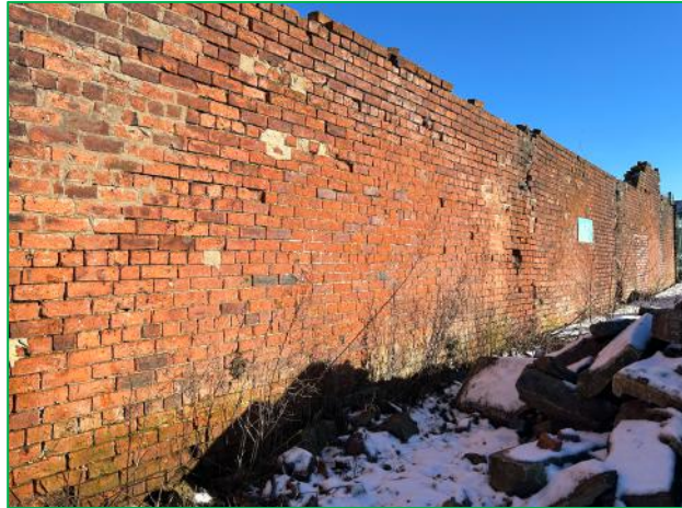
The wall along the northern boundary
