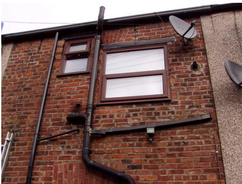
Rear elevation – view at first floor.
