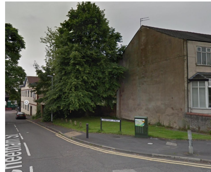
View from A576 down Cheetham Street towards frontage of site
