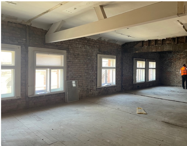
Interior After Strip Out
