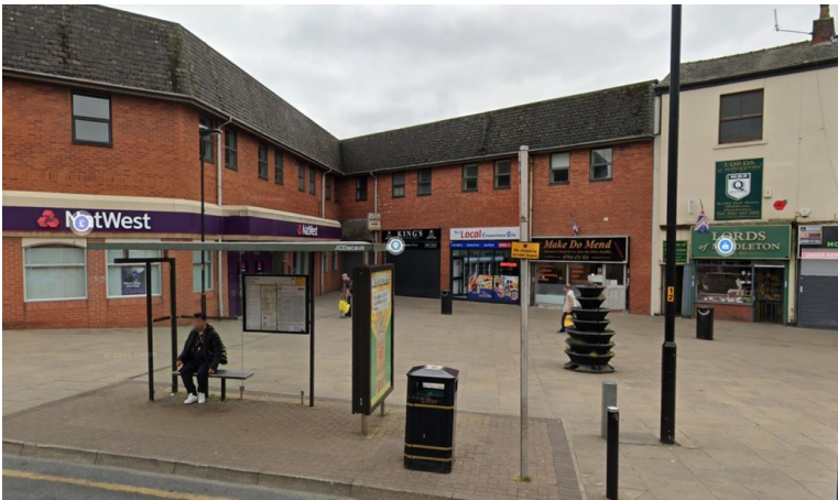
Street View of Building
