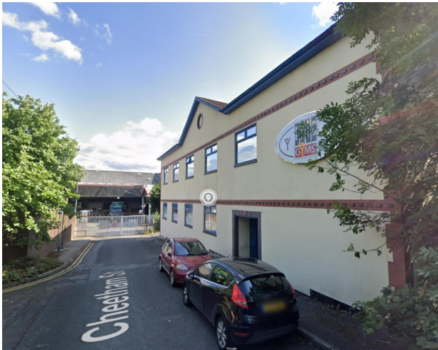
Front Elevation showing existing building materials
