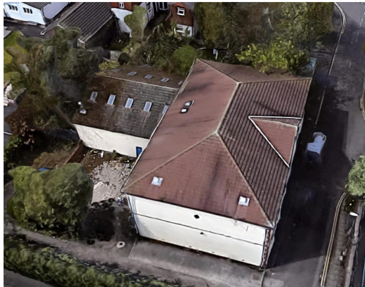
Aerial View of the Existing Building on the site
