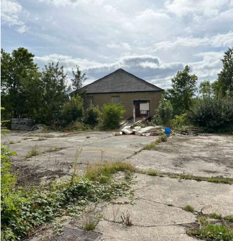
Figure 4.6: Rear Elevation of the Former Milnrow Reform Club (August 2025)
