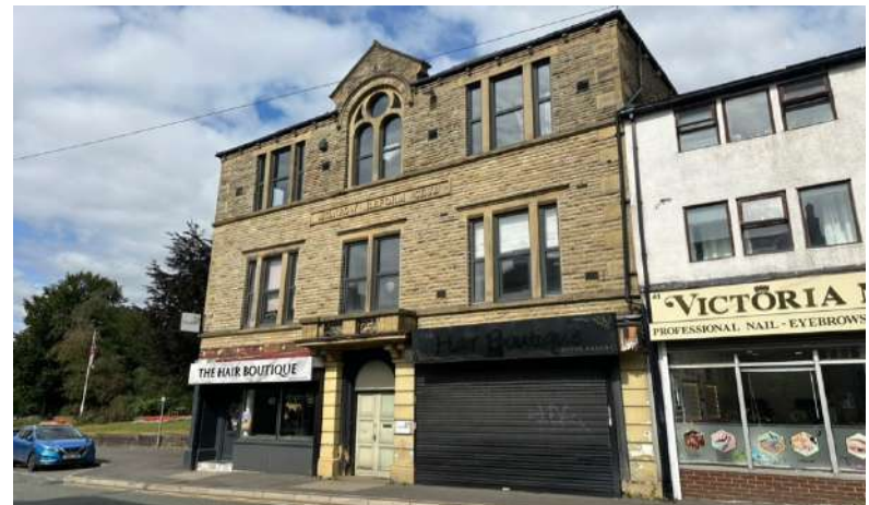
Figures 3.2 & 3.3: Northern and Southern Components of the Application Site (August 2025)
