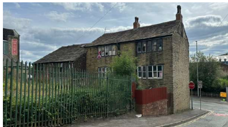
Figure 4.10: Rear of 45/47 Dale Street (August 2025)
