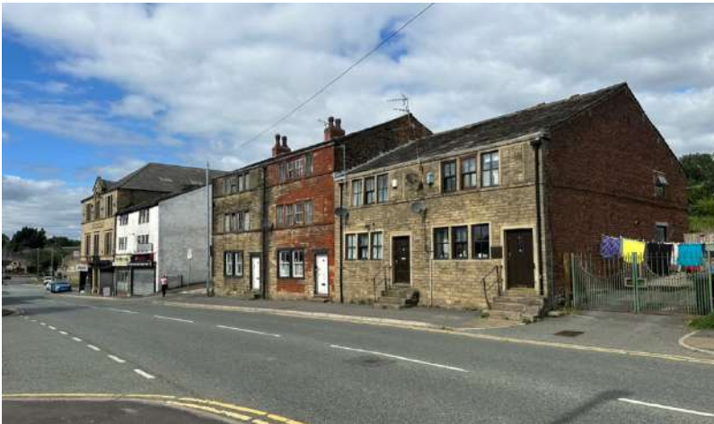
Figure 4.7: View of the Former Milnrow Reform Club (August 2025)
