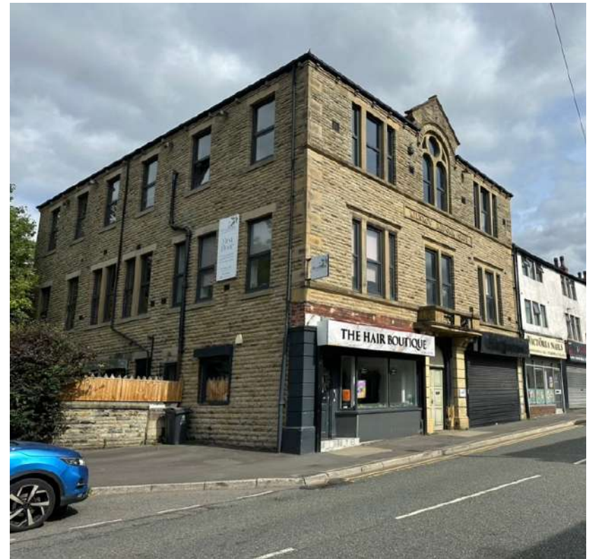
Figure 4.5: Side Elevation of the Former Milnrow Reform Club (August 2025)
