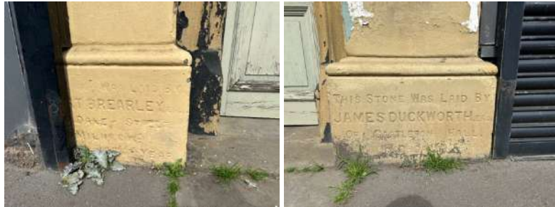
Figures 4.3 & 4.4: Stones to Main Entrance (August 2025)
