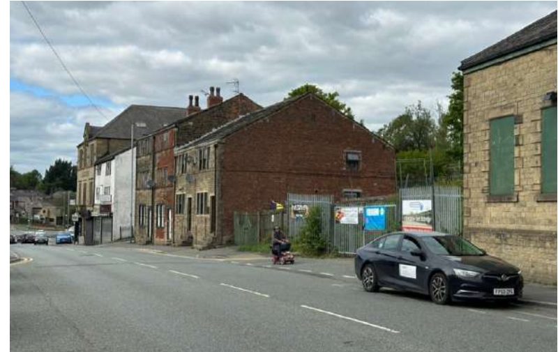
Figure 4.12: View along Dale Street (August 2025)
