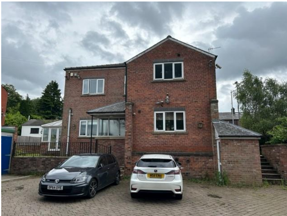
Rear view of property – proposed extension on the left hand side of the image.
