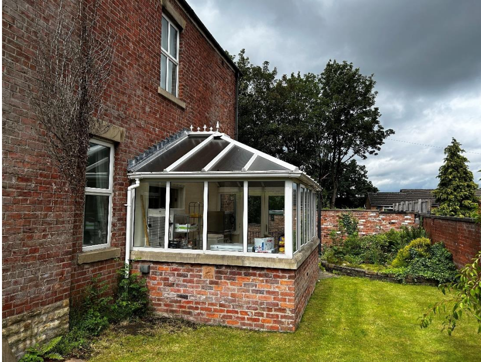
Side elevation – conservatory to be demolished.
