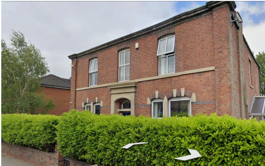
Front elevation to Rochdale Road East.
