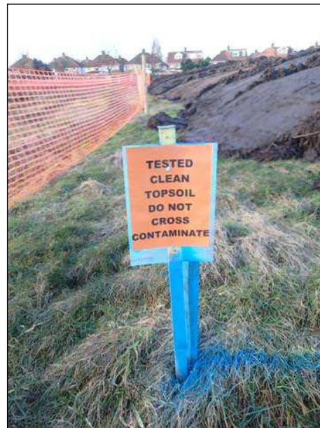
Photograph 4: Example of good stockpile management with warning signs and fencing to prevent accidental cross-mixing.
