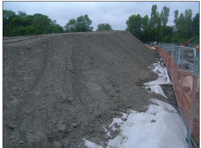
Photograph 2: Example of good stockpile management with soils placed on geotextile with fences to prevent accidental cross-mixing.
