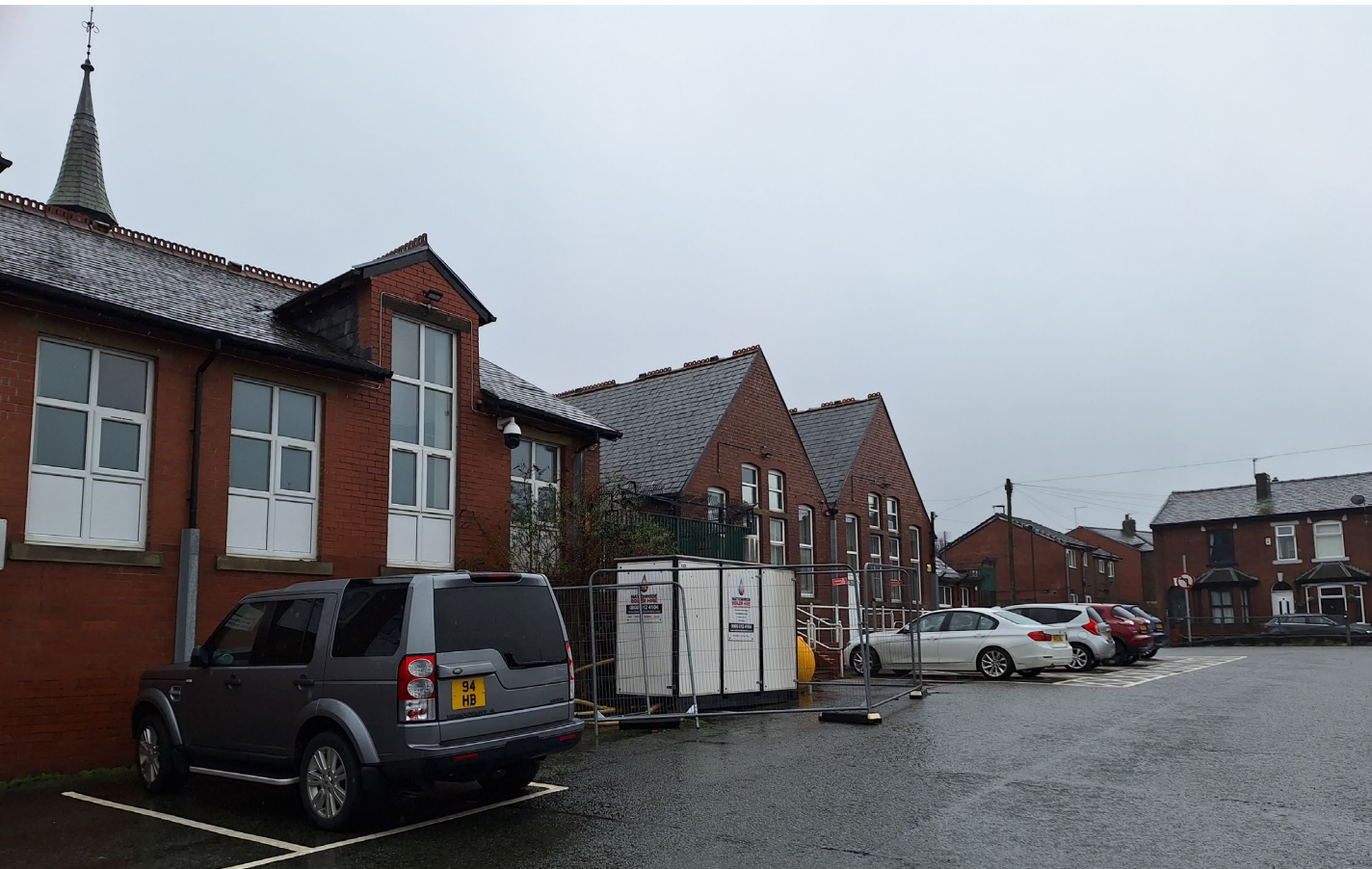
Photos of West Elevation showing existing temporary boiler enclosure (Feb 2024)
