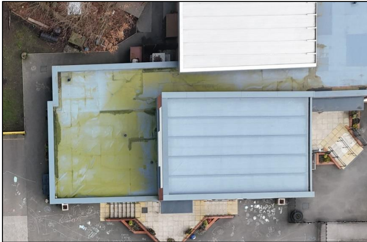
Photograph 8 showing the part of the building to be extended
