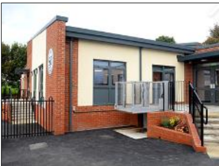
Photograph 3 showing the newer portion of the building.
