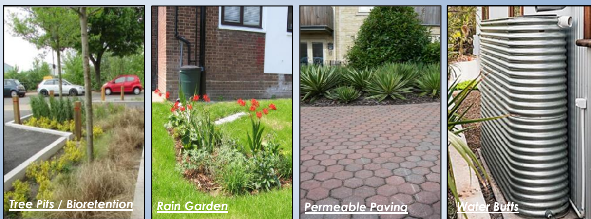
Figure 3: SuDS Photographs (SusDrain, 2012)
