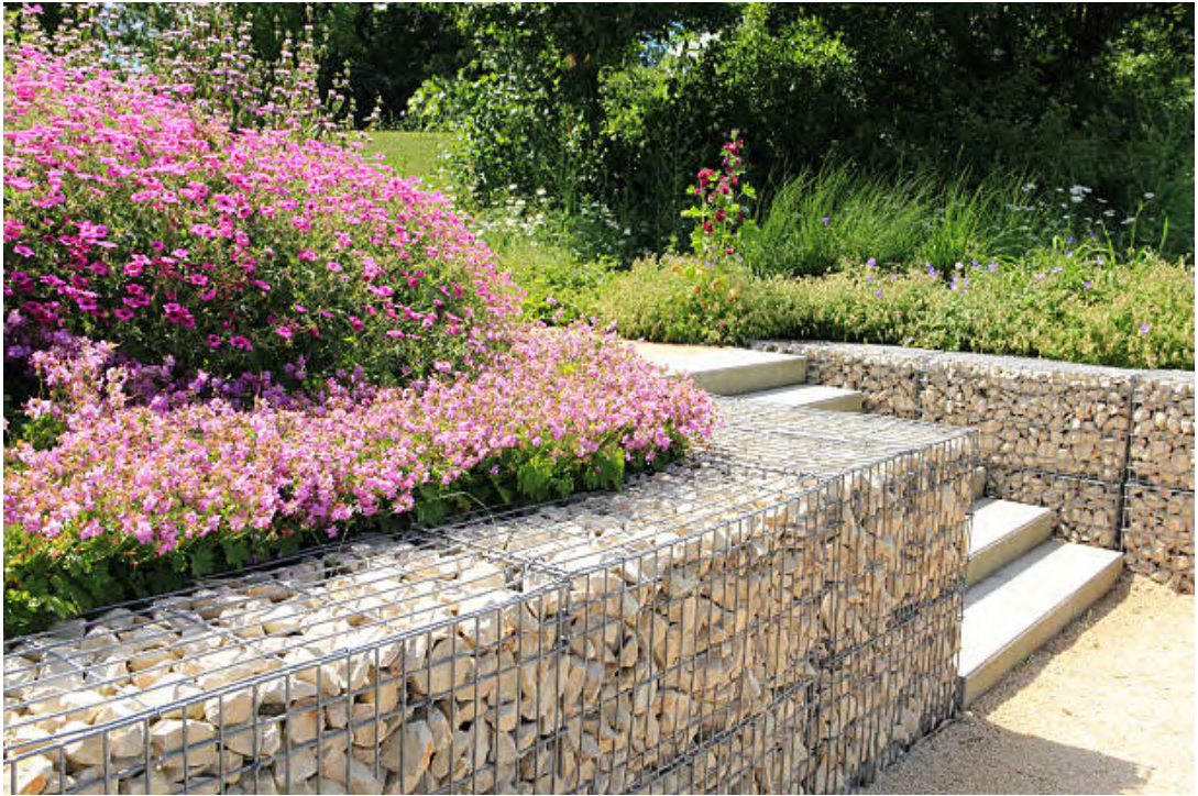
1M high gabion basket retaining walls
