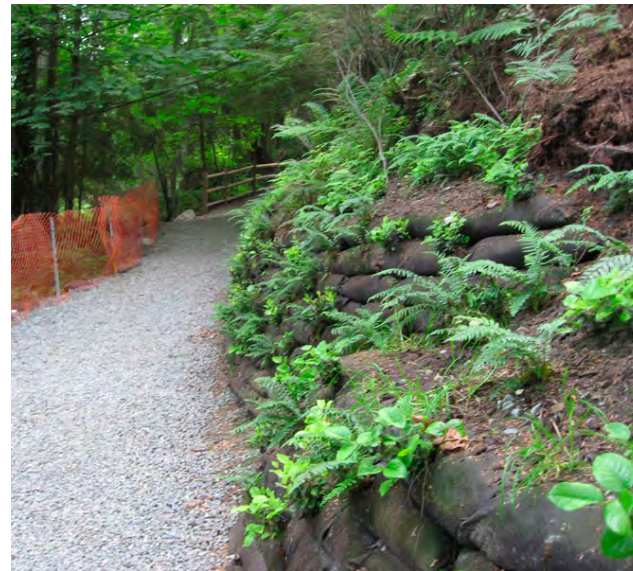
Flex MSE shortly after construction
