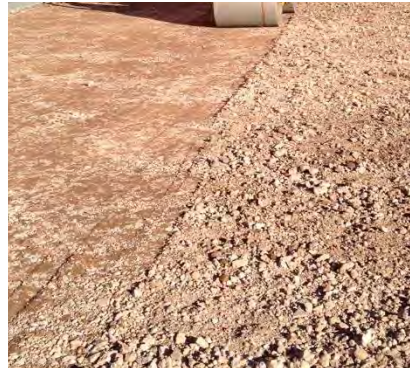
Compacted MOT Type 1 aggregate
