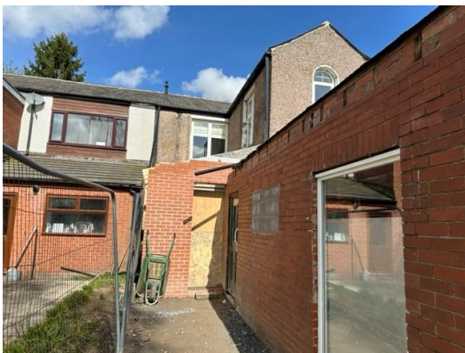
Figure 2.4: Close up of rear extension
