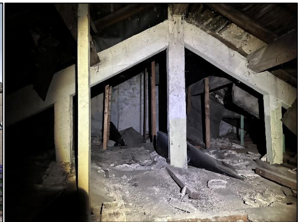
Figure 4: The roof void within the building.
