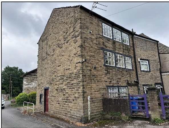
Figure 3: The northern elevation of the building.
