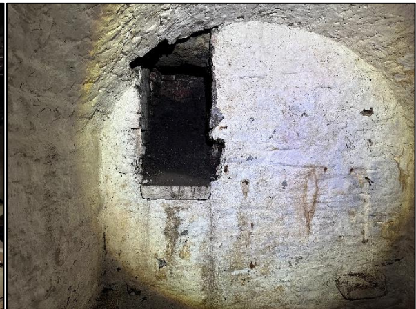
Figure 11: The cellar below the building.
