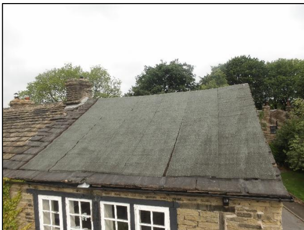
Figure 8: The felt covered roof of the building.
