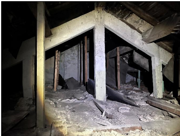
Figure 10: The roof void within the building.
