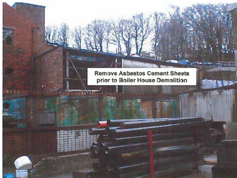
Asbestos Cement Sheets to be removed prior to Boiler House Demolition
