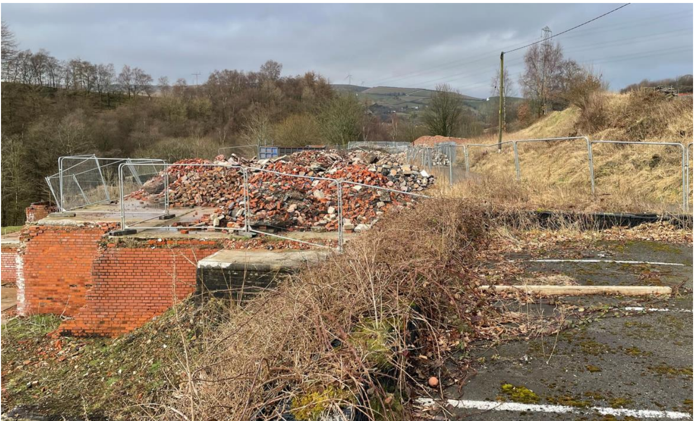
Demolition materials separated for removal.
