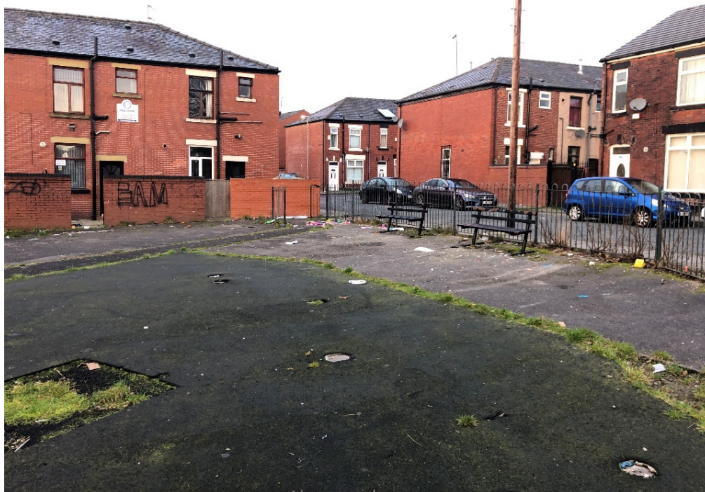
Photograph 3 – The former children's playground on Block A.
