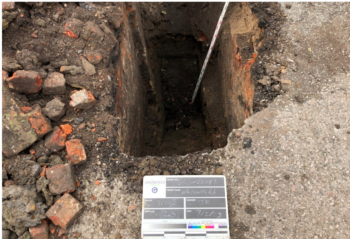
Photograph 8 – TP105 Showing basement walls
