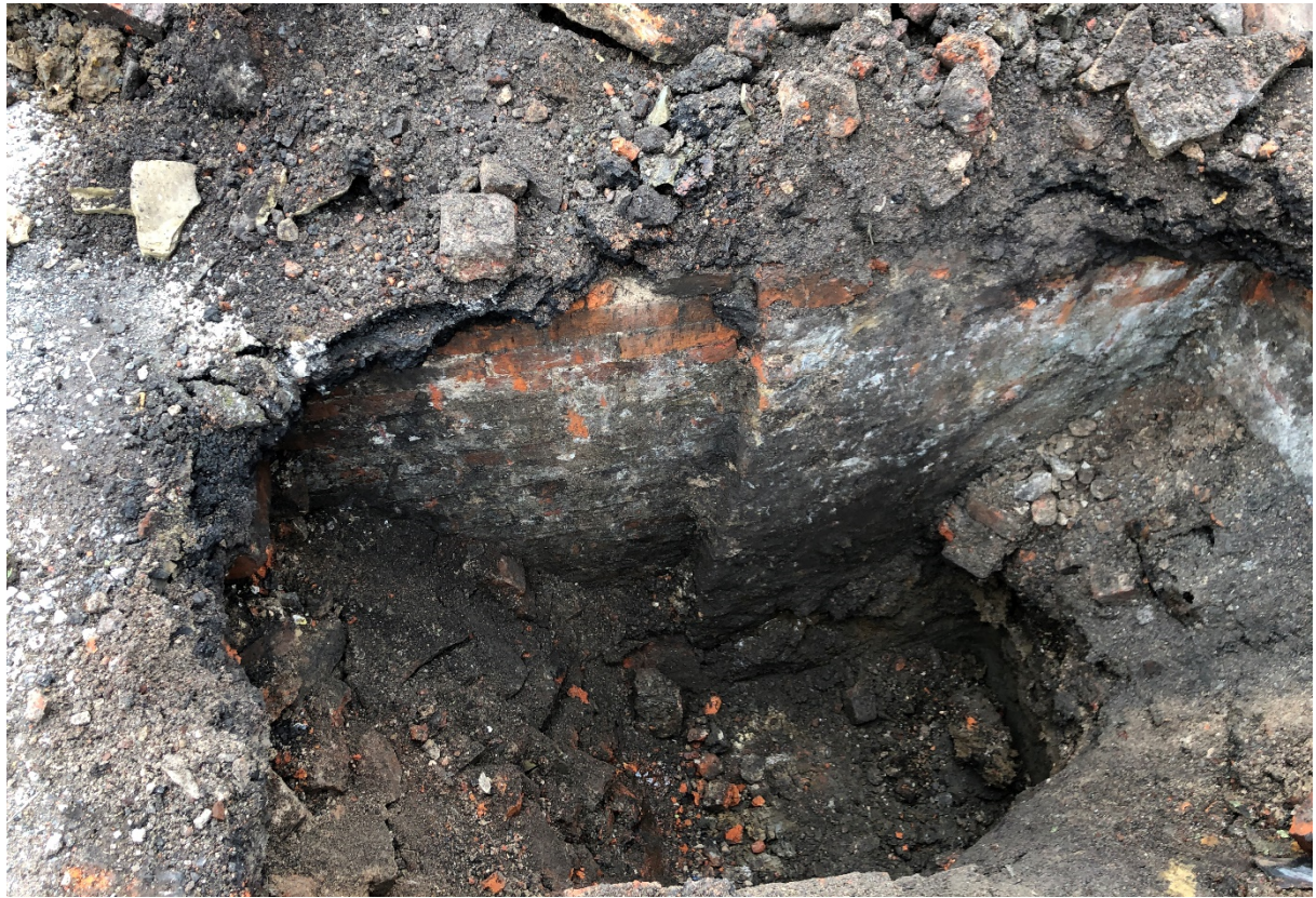
Photograph 9 – Brick wall in side of TP105
