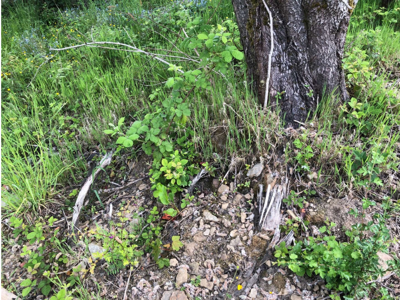
Root damage and destruction to T1.
