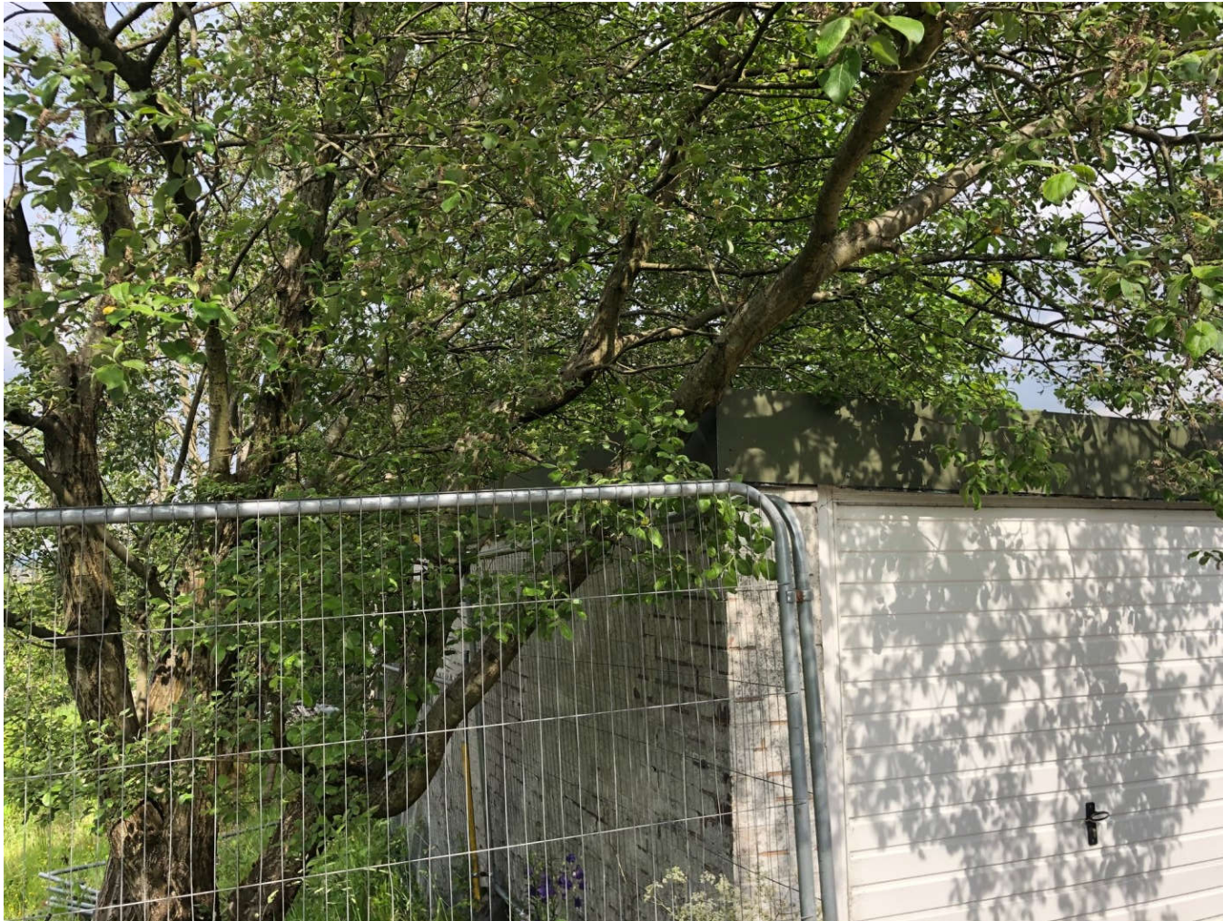
Overhanging canopy of T4 across garage.
