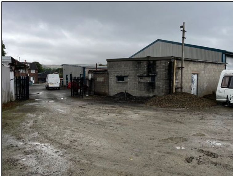
General view to the north west towards the existing partially demolished structure at the site
