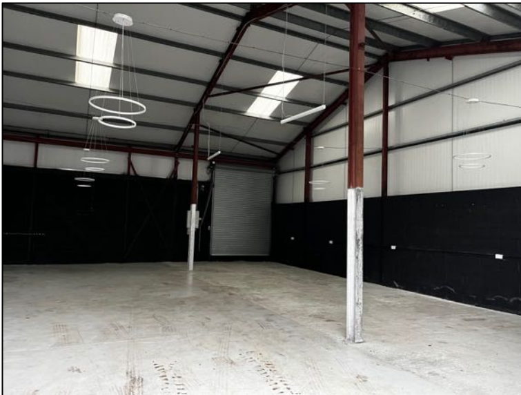
View of existing development immediately north of the development site showing interior of unit with concrete slab
