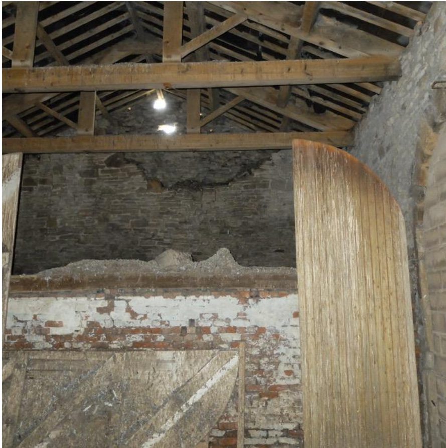
Photo. Threshing barn doors
