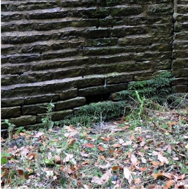
Photo. Air vent in front elevation
