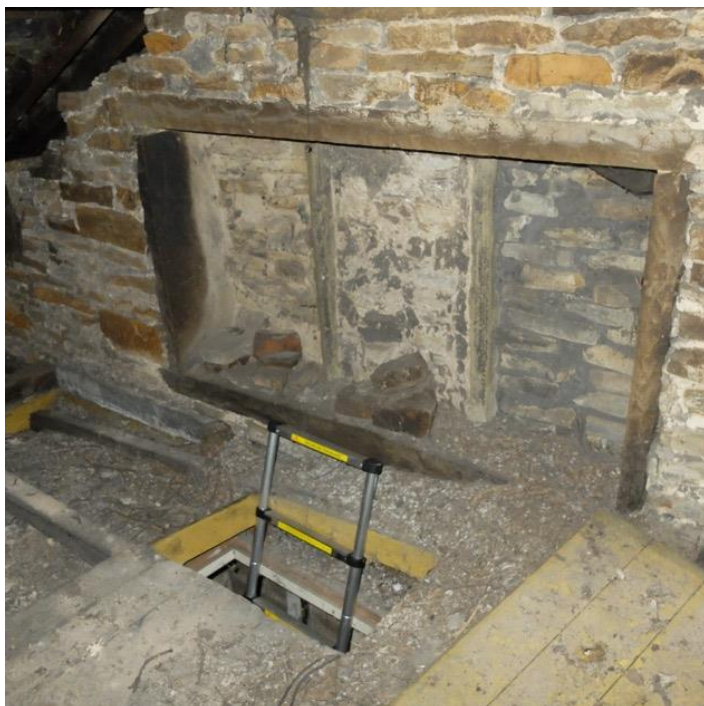
Photo. Infilled window to east gable.
