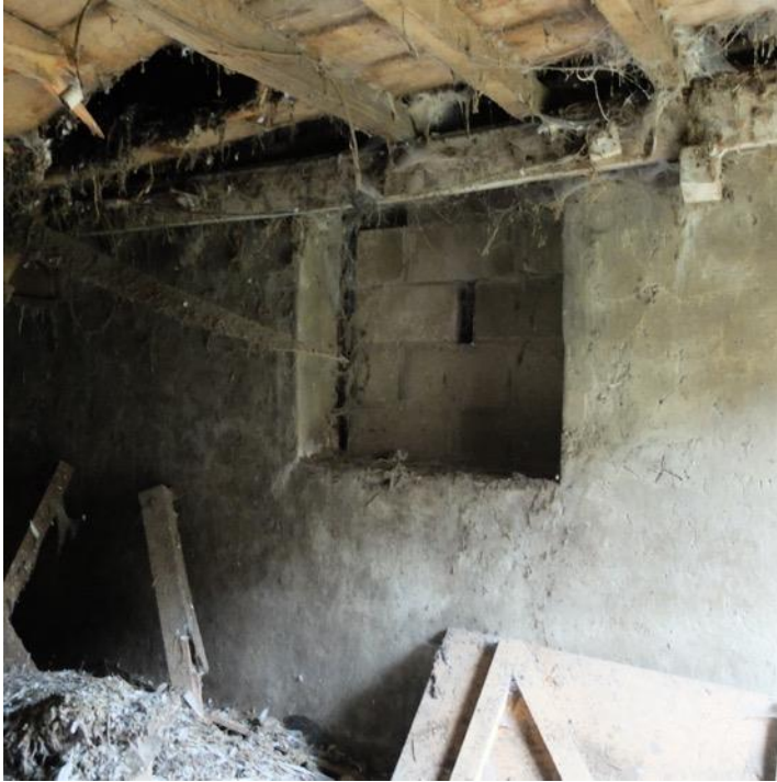
Photo. Loft floor above left hand section of the barn
