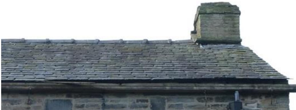
Photo. Diminishing coursed slate roof to farmhouse
