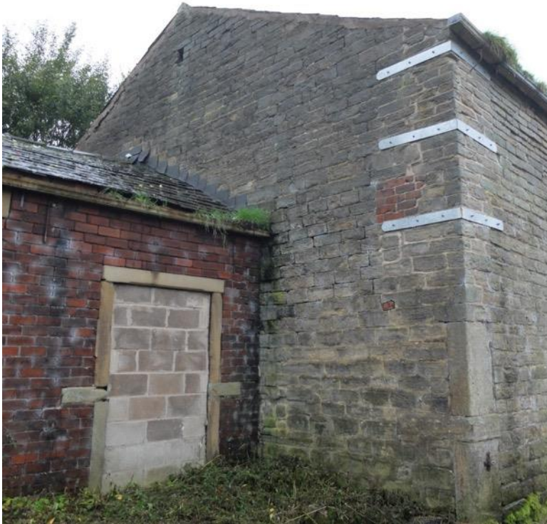
Photo. Old bricked up flue and corner strapping
