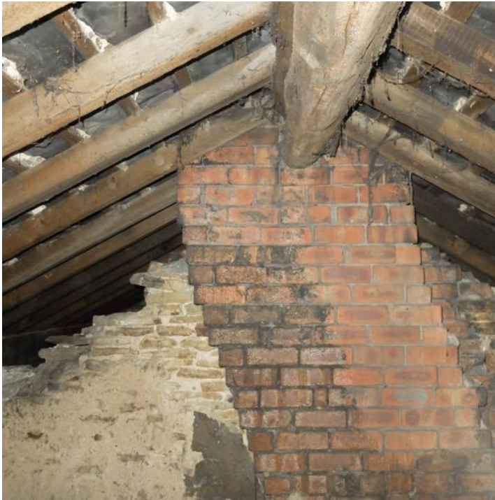
Photo. Newer brick chimney to Space R2, log ridge, which is original roof structure, note old plaster to walls
