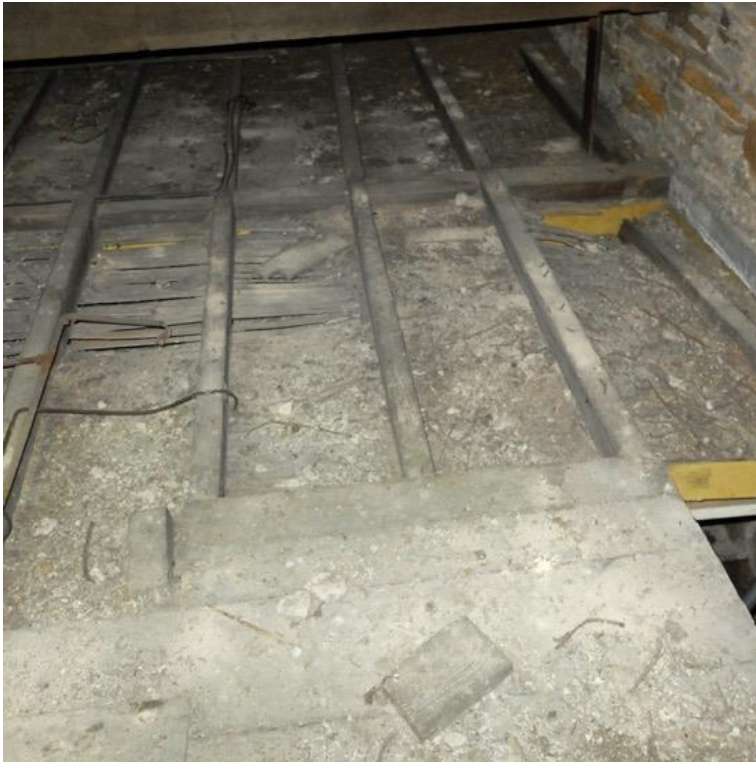
Photo. Ceiling joists with old nails indicating floor boarding.
