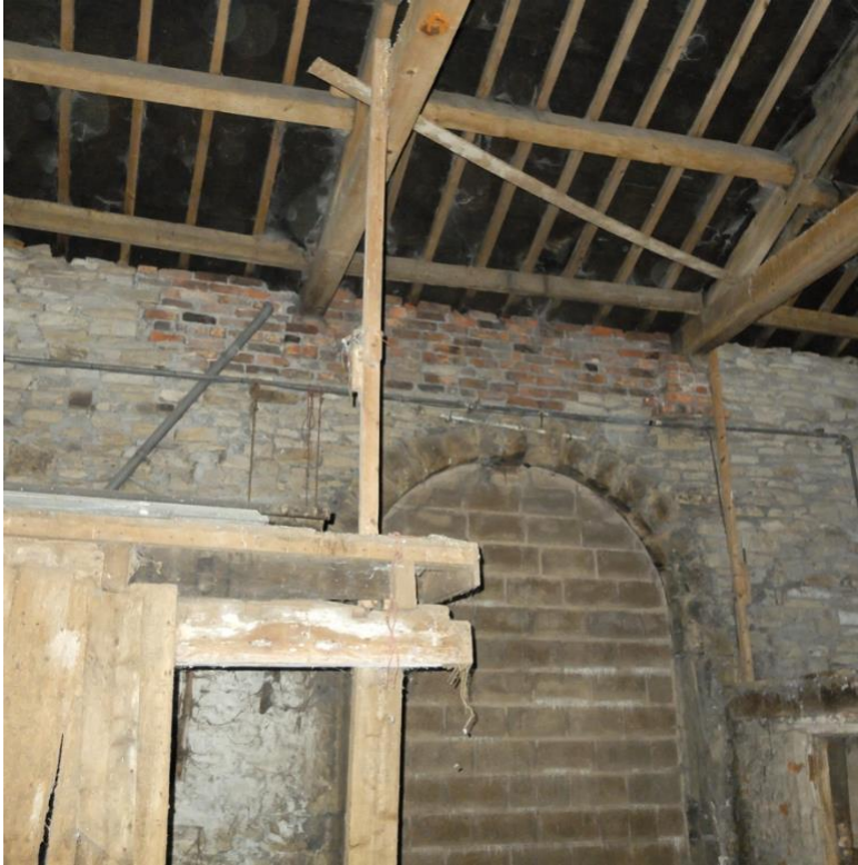
Photo. Rebuilding inner leaf in. brickwork
