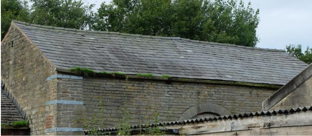
Photo. diminishing coursed slate roof over barn
