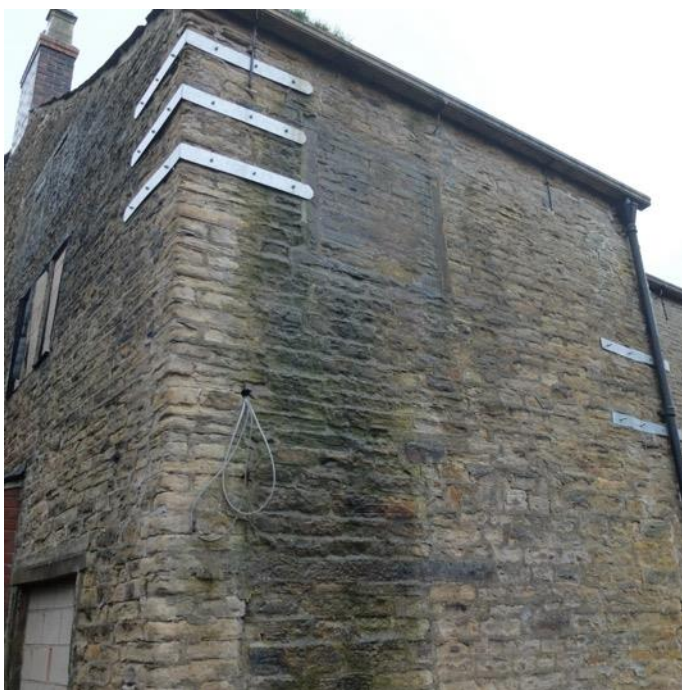
Photo. Corner straps to high level.
