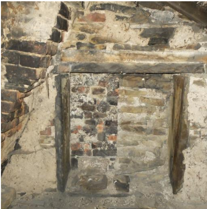
Photo. Old window infilled with masonry.
