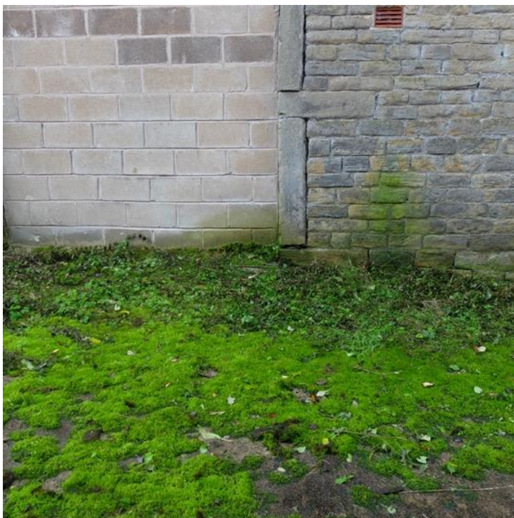
Photo. Repacking of threshing door reveals
