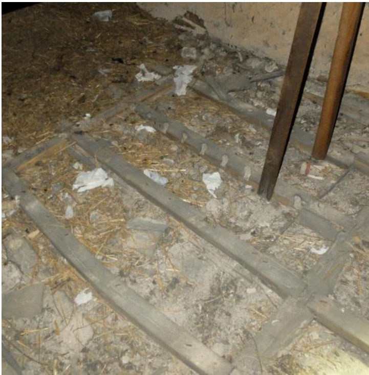
Photo. Old ceiling trap in location of hangers above room F.04
