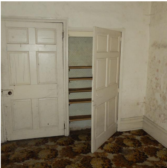
Photo. Original doors to farmhouse Room G.03
