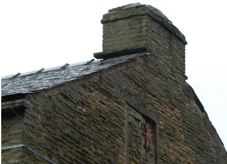
Photo Stone Chimney with weathering course to left gable.
