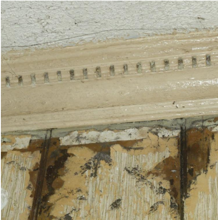
Photo. Timber partition with timber cornice
