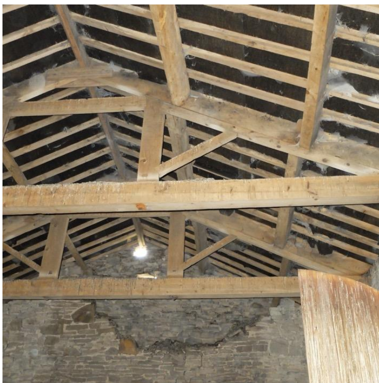
Photo. Queen post roof structure of barn (considered 1900s)
