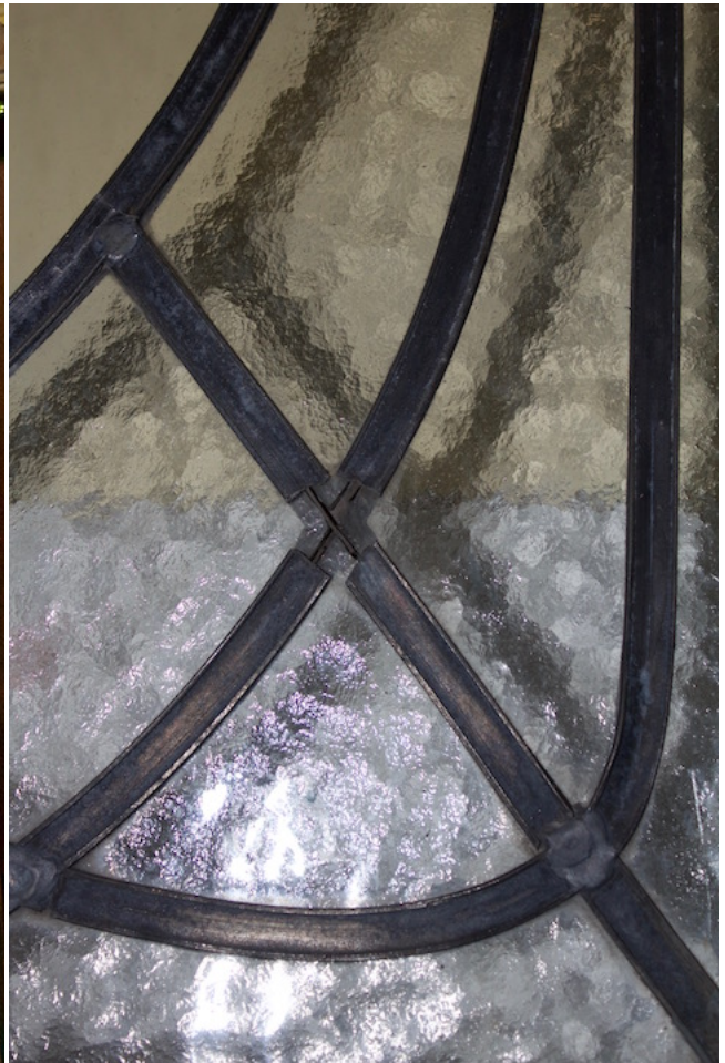
Example of broken solder
