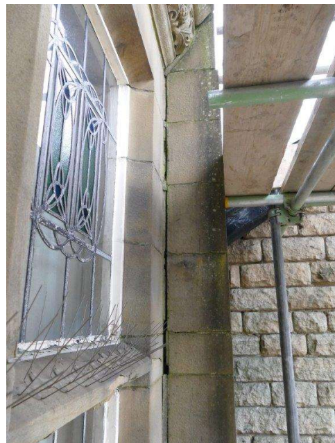
The south pier and finial has a distinct lean to the south which has further opened the joint to the gable panel
