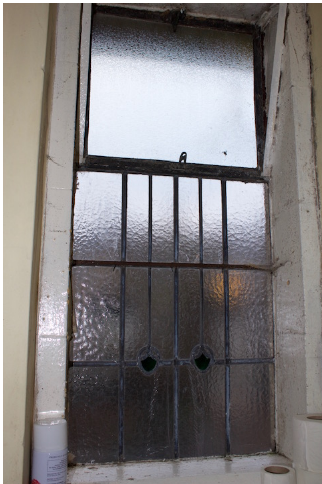
Toilet window internal
