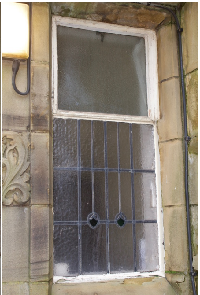
Toilet window external
