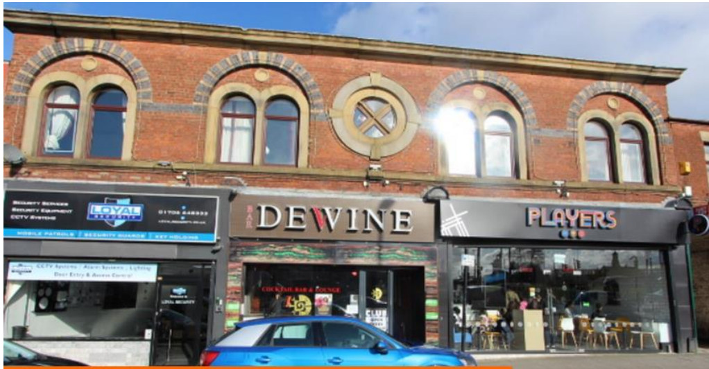
Photo above shows the shopfront as existing.
