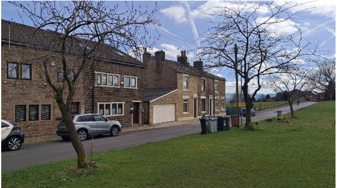
Photo 7: No. 143 Syke Road with two of the listed cottages to left
