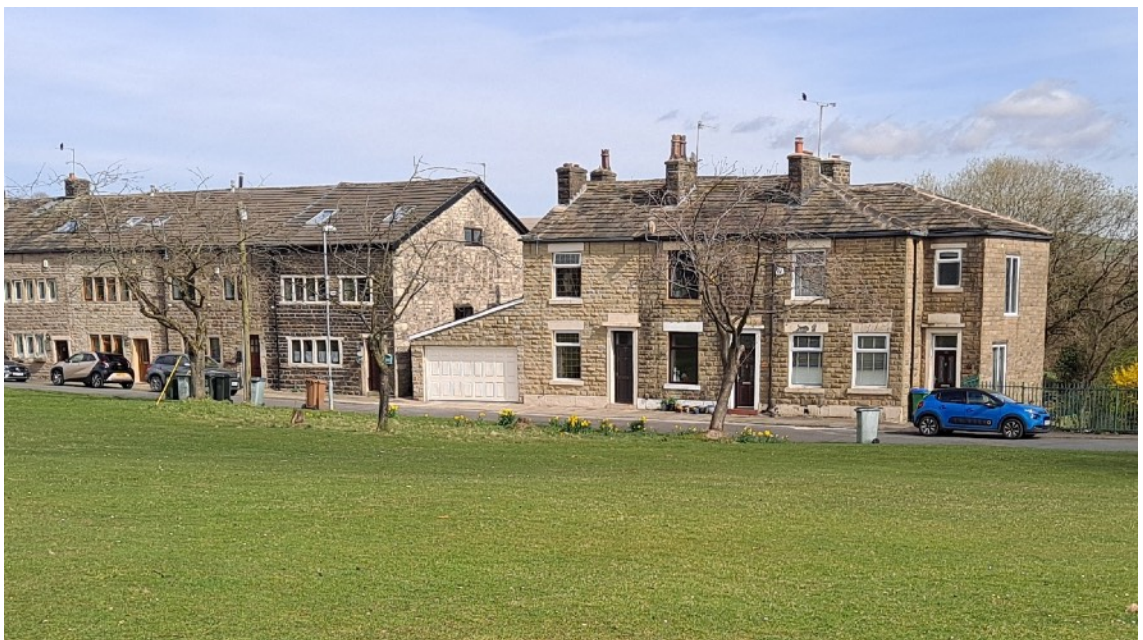
Photo 8: Nos 141-143 Syke Road with listed cottages to left
