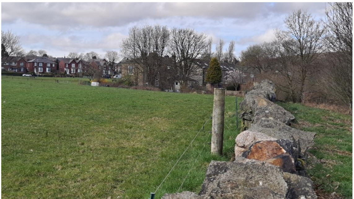
Photo 4: Looking to the rear of the cottages from the south-east
