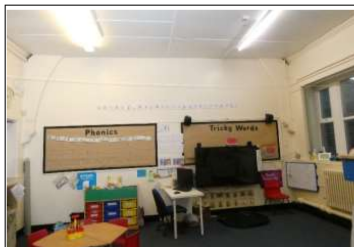
Partition and Roof Truss With Suspended Ceiling
