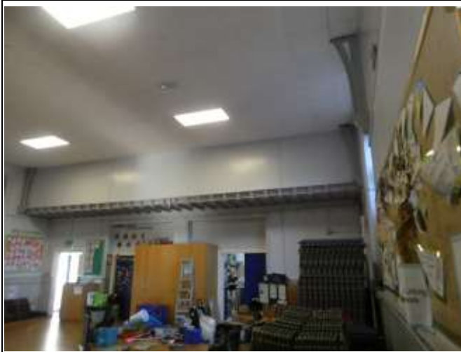
Hall with Suspended Ceiling
