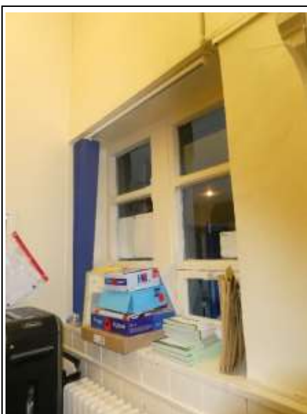
Window at the Entrance Lobby
