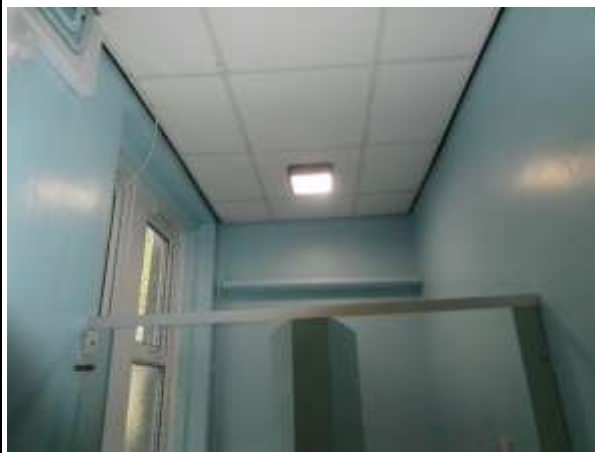
Boys WC with Suspended Ceiling
