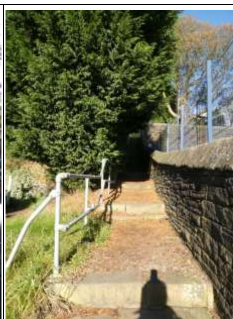
Looking North – Stone Steps to the West of the Building
