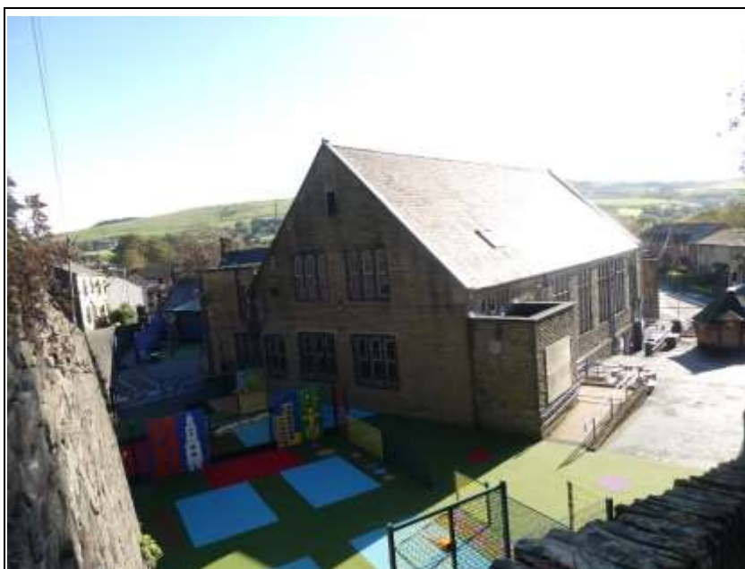
Looking Southeast Towards the Building from the Top of the Stone Steps to the West
