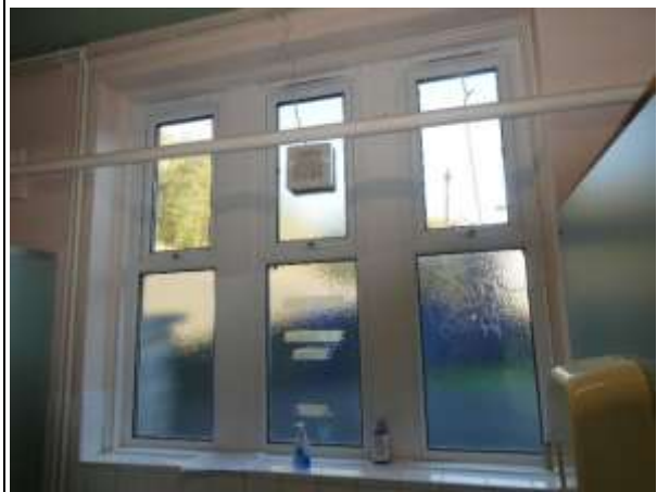
Window at the Northeast Elevation – Girls WC
