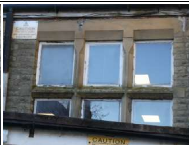
Original Mullion Windows Above Main Entrance
