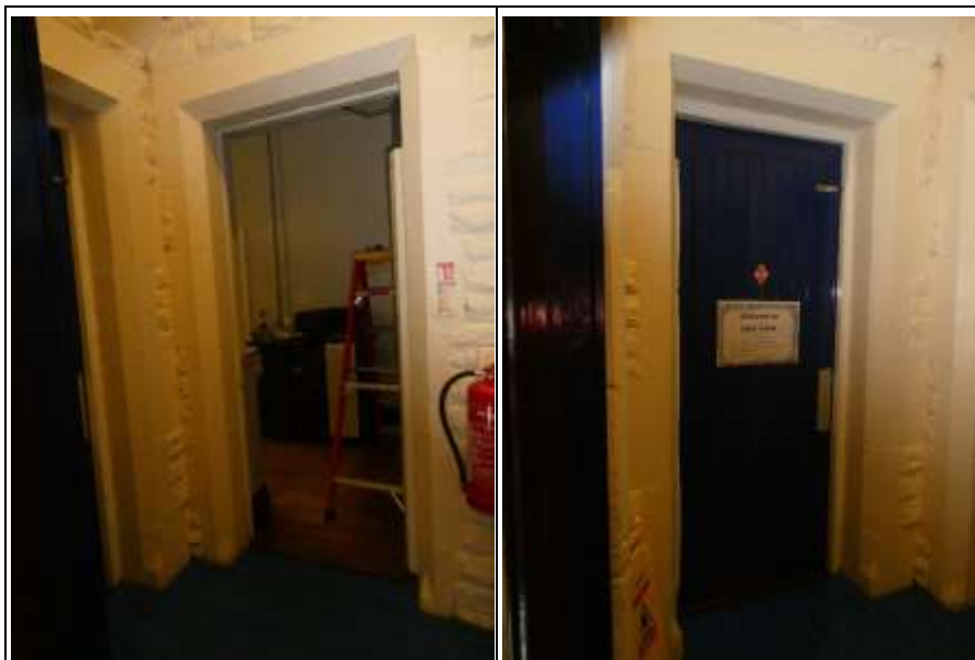
Doorway off Hallway – South of the Head's Office
