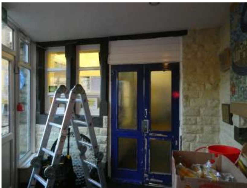
Door Leading to Offices
