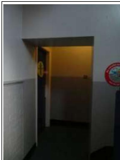
Corridor Leading to Boys WCs
