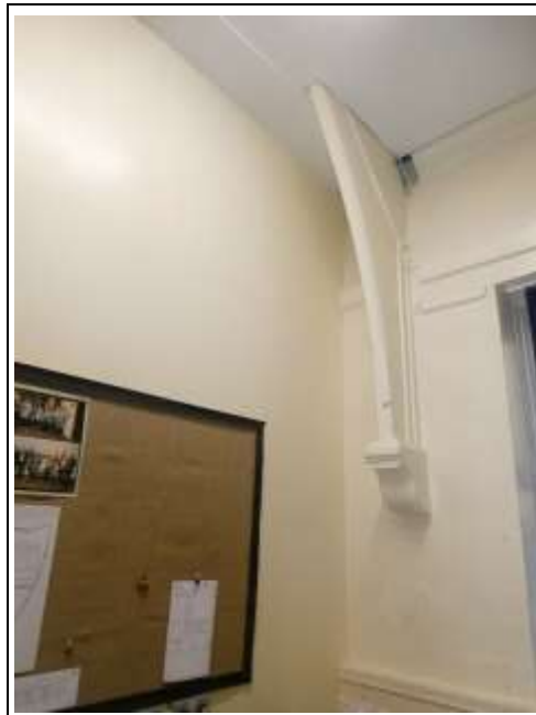
Bracket and Base of Roof Truss
