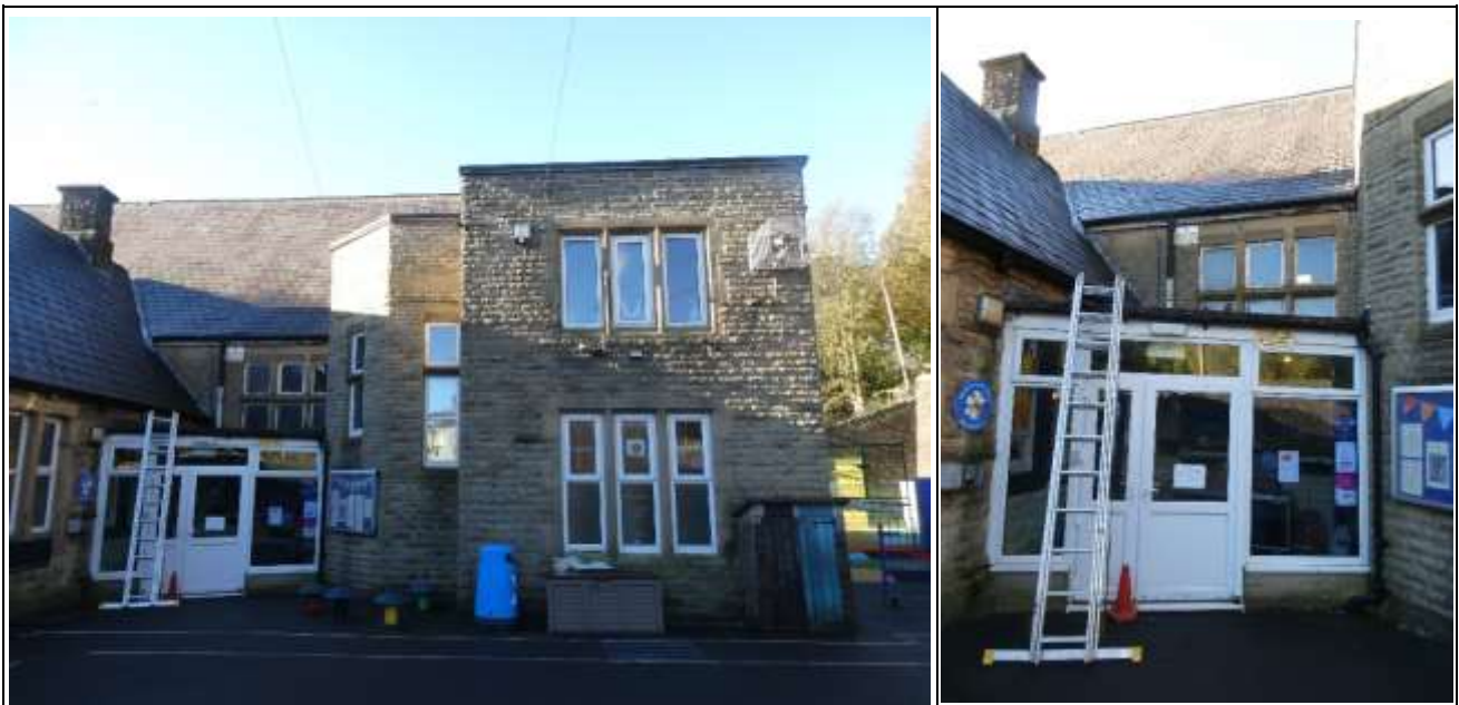
Existing Main Entrance with Flat Roof
