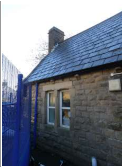
Section Located to the Southeast Corner
