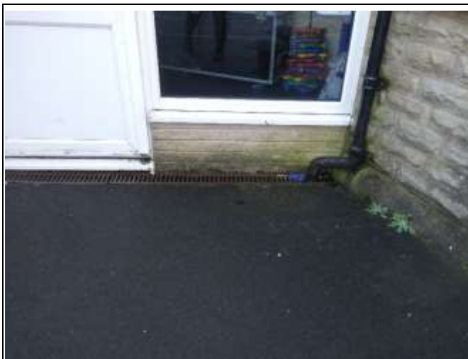
Faux Stone Base of Entrance Lobby
