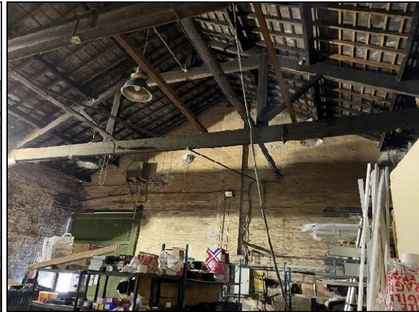
Figure 23: The interior of Building 3.
