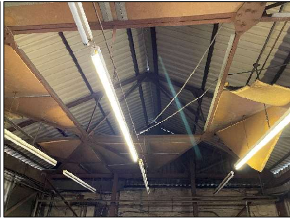
Figure 19: The interior of Building 2.
