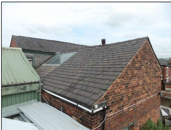
Figure 3: The rear (eastern) elevation and roof of Building 1.
