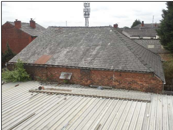
Figure 9: The roof of Building 3.
