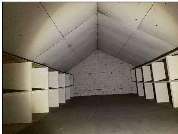
Figure 4: The lined loft space within Building 1.
