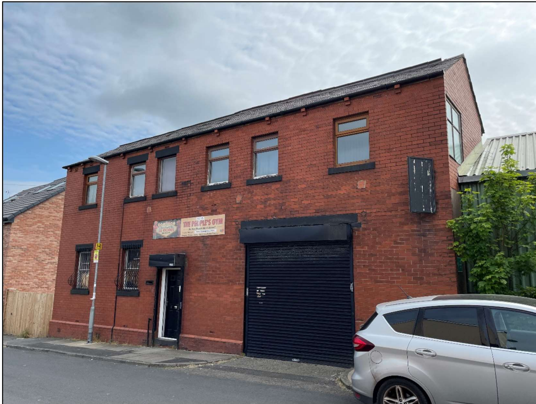
Figure 2: The front (western) elevation of Building 1.
