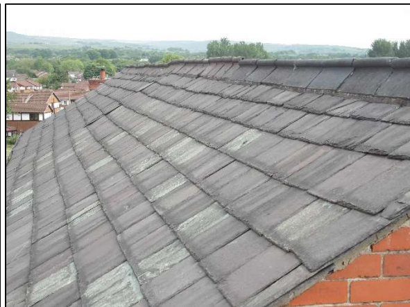
Figure 17: Looking along the roof of Building 1.
