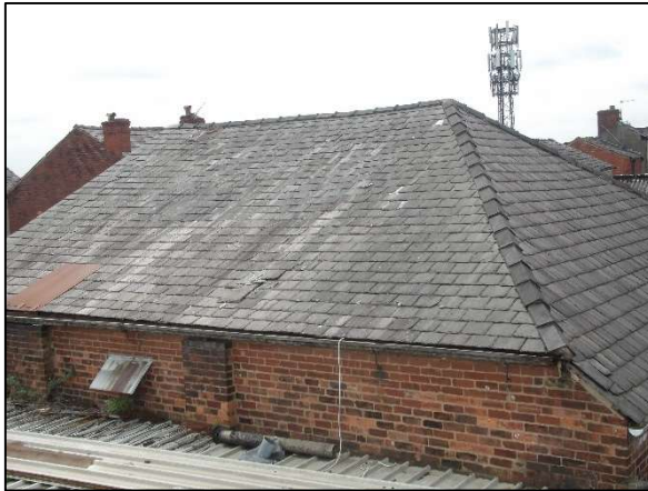
Figure 22: The roof of Building 3.
