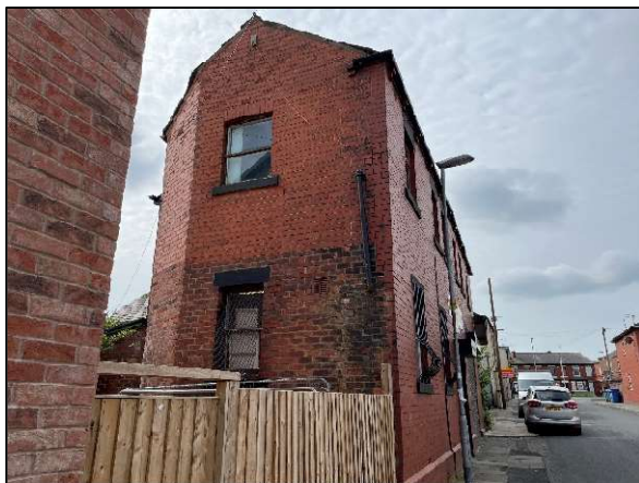
Figure 12: The northern elevation of Building 1.
