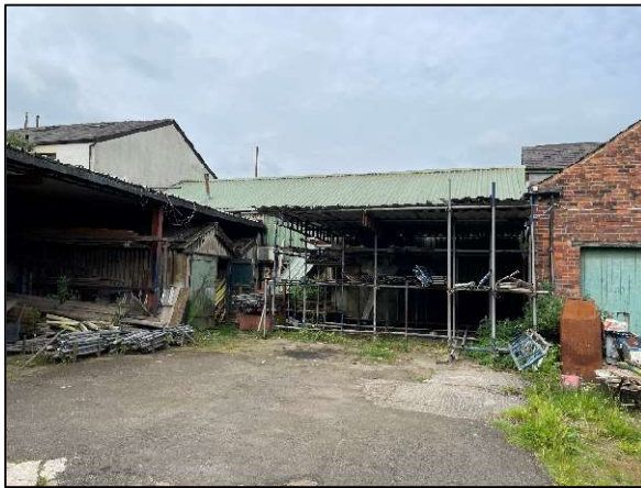
Figure 6: The rear (western) elevation of Building 2.
