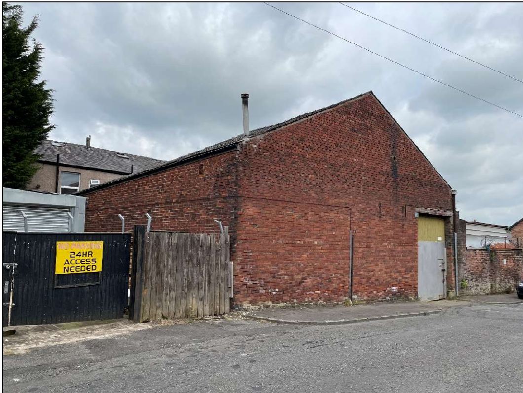
Figure 8: The eastern elevation of Building 3.
