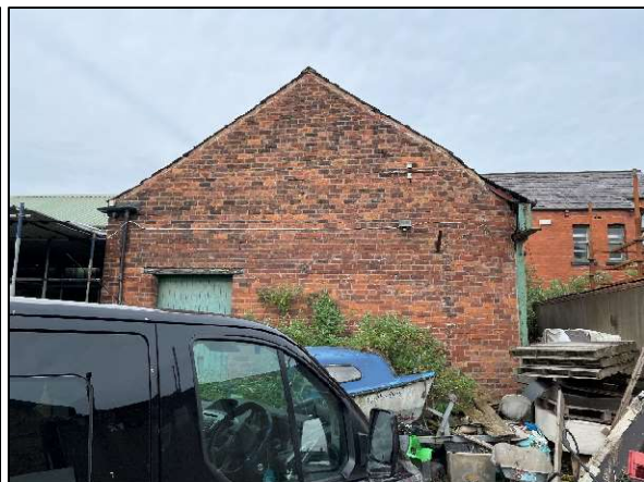
Figure 13: The eastern elevation of Building 1.
