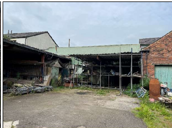
Figure 25: Areas of metal racking behind the buildings.
