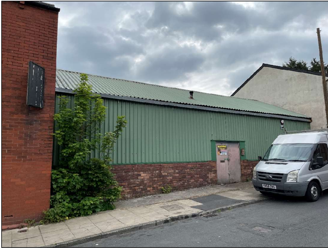
Figure 5: The front (western) elevation of Building 2.
