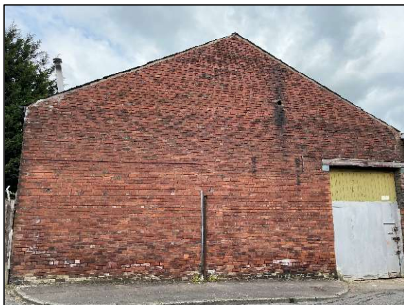
Figure 20: The brickwork of Building 3.
