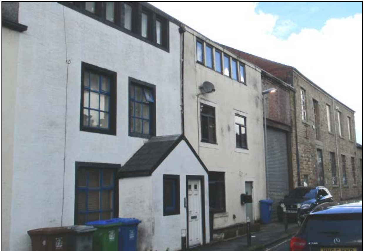
4. The adjoining cottages have however retained their domestic appearance
