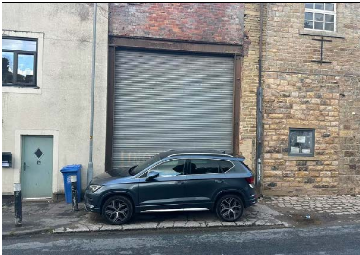
3. Front elevation is dominated by the loading bay door
