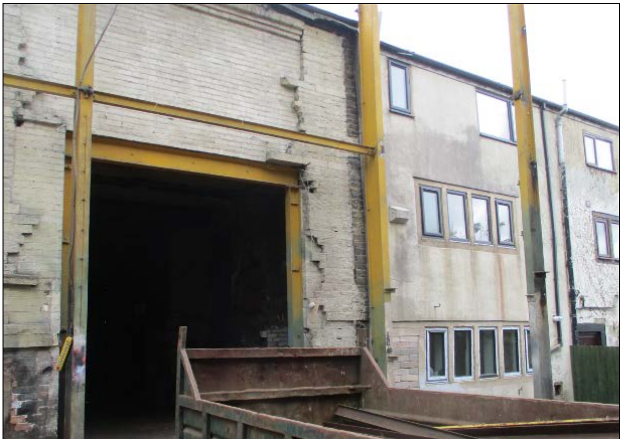
5. Similar opening on the rear elevation
