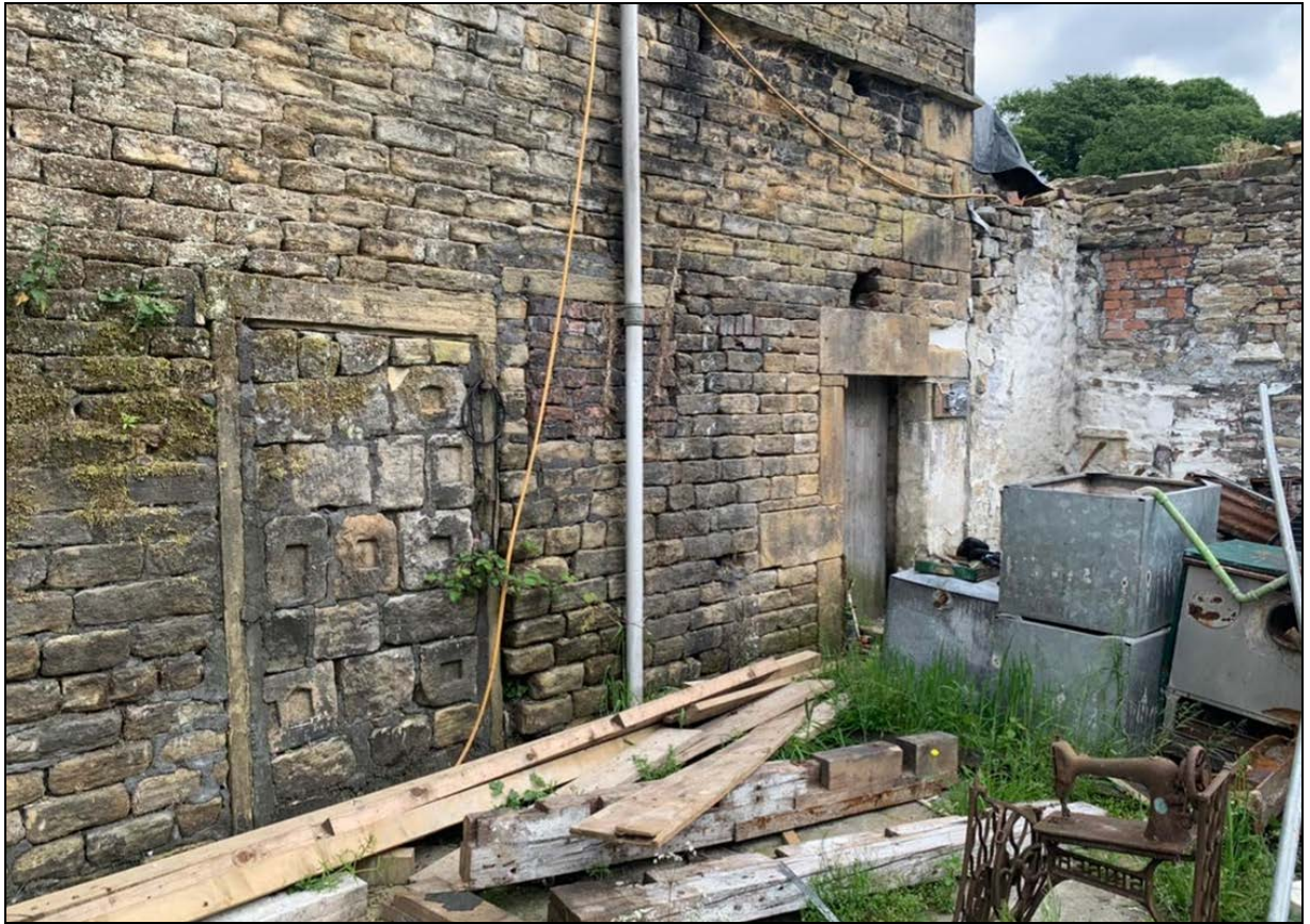
6. Doorways to the third bay, nearest one inserted later and now blocked
