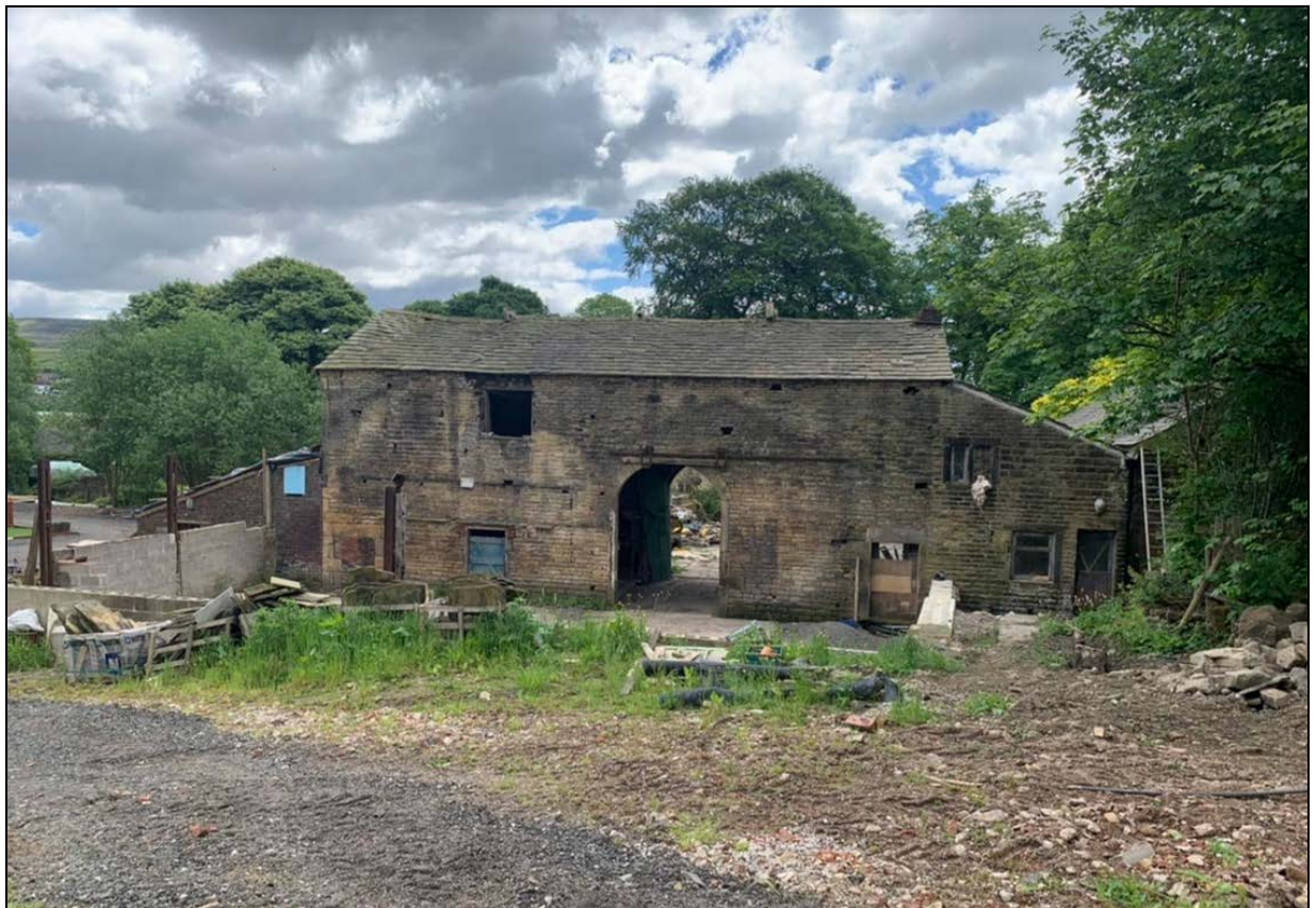
2. The barn viewed from the rear
