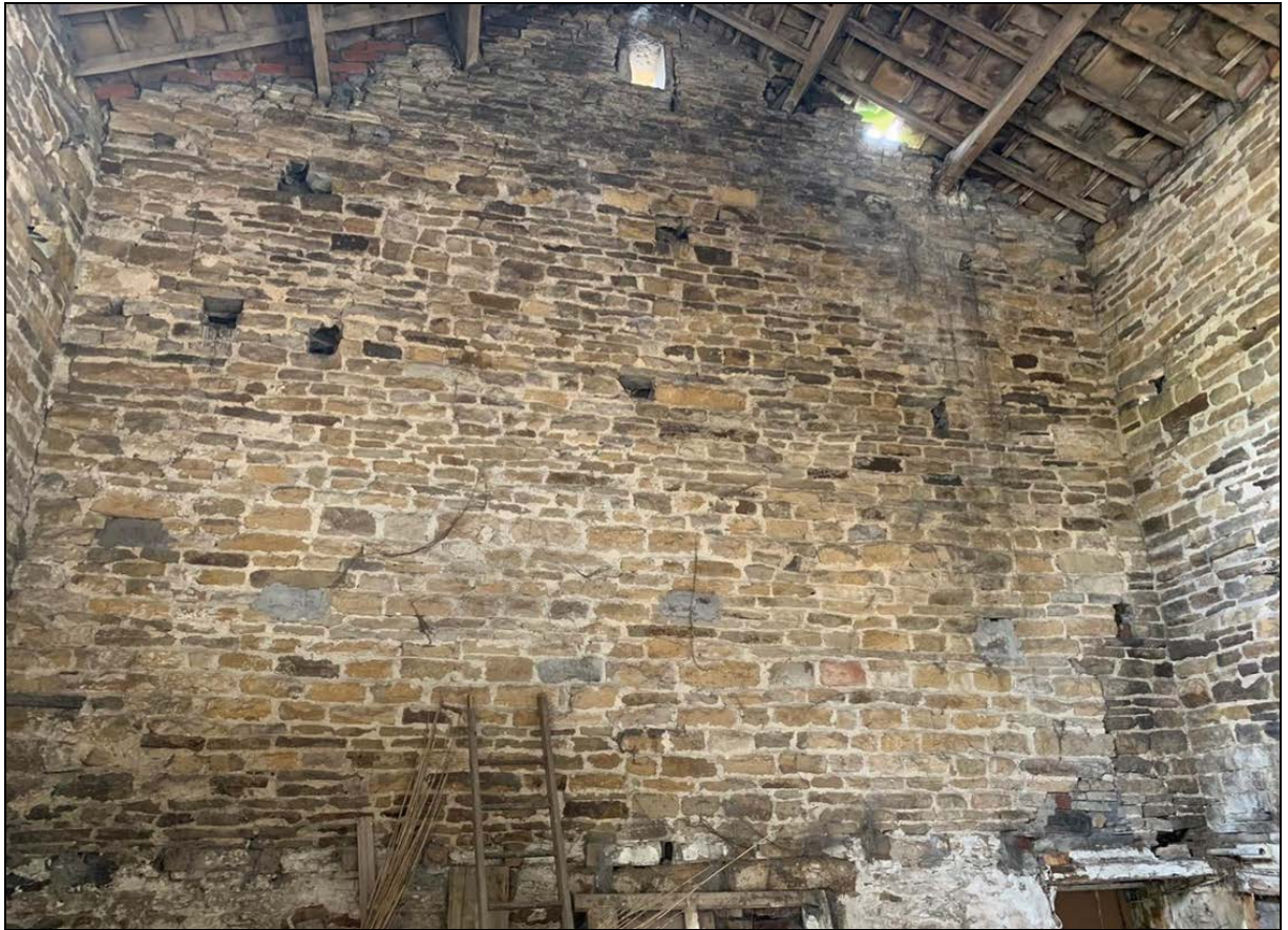
10. The third bay of the barn is open, but hayloft door indicates a floor once existed
