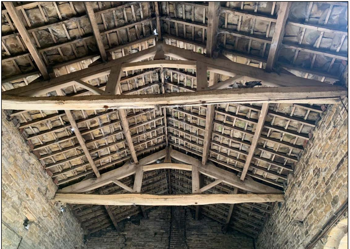
9. Kingpost trusses machine-cut, but with reused tiebeams
