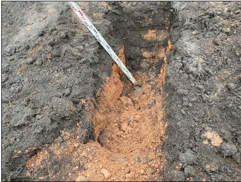
View of Plot 16 rear garden excavated to a depth of 0.80m exposing geotextile membrane at base.
