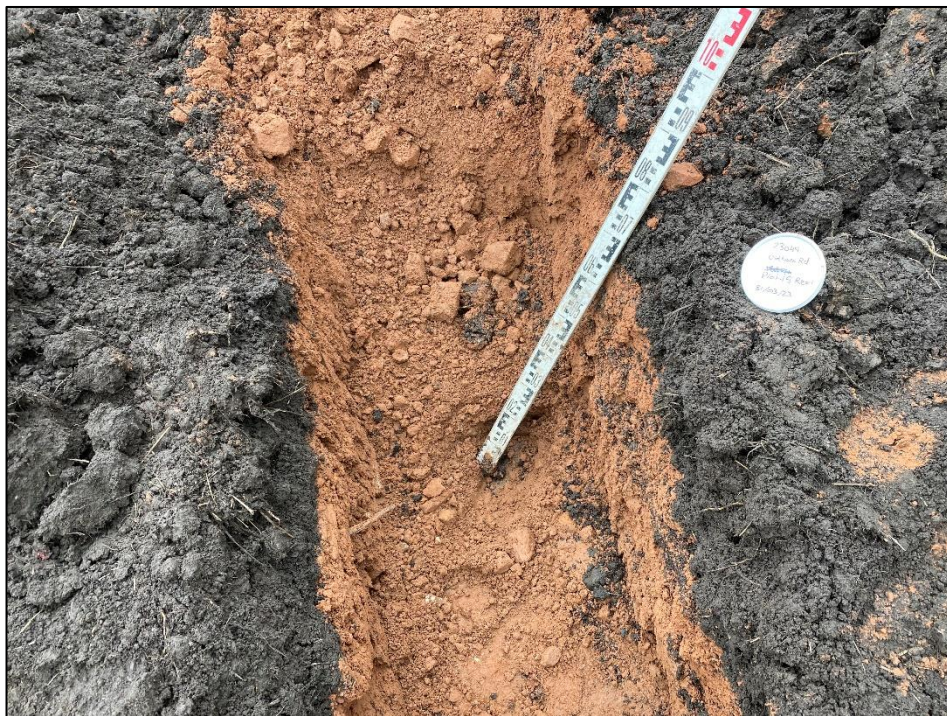
View of Plot 15 rear garden excavated to a depth of 0.85m exposing geotextile membrane at base.
