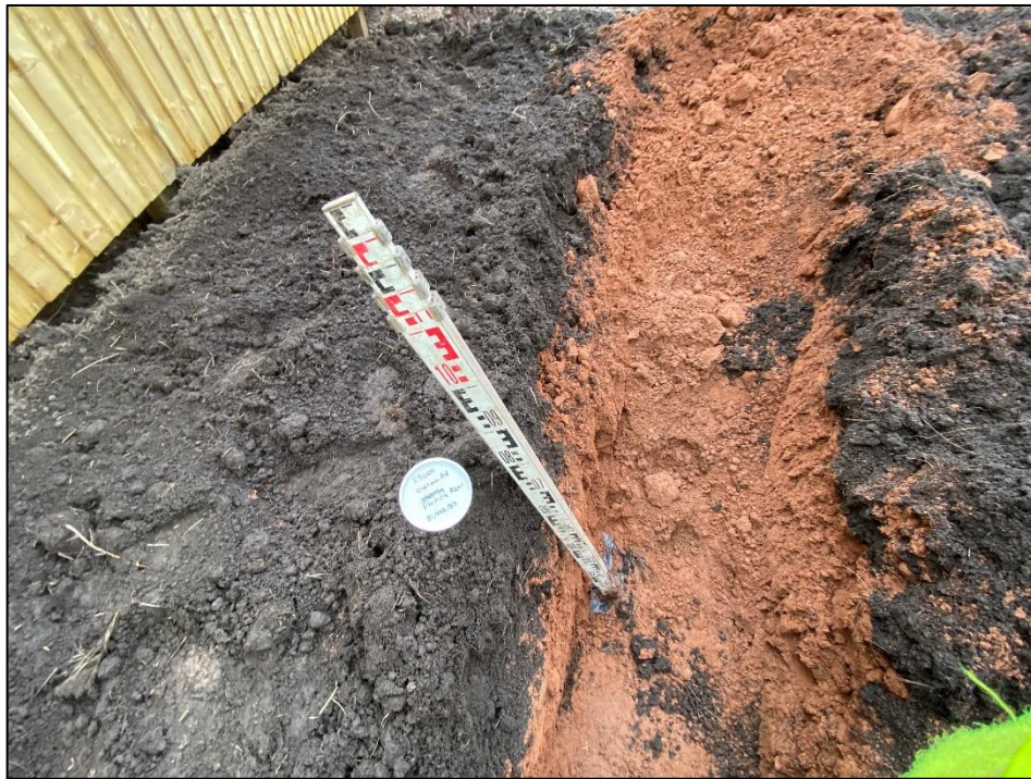
View of Plot 14 rear garden excavated to a depth of 0.80m exposing geotextile membrane at base.
