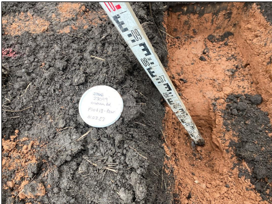
View of Plot 13 rear garden excavated to a depth of 0.80m exposing geotextile membrane at base.
