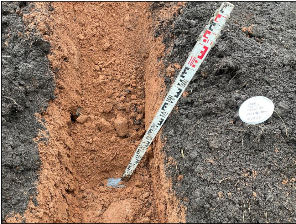
View of Plot 10 rear garden excavated to a depth of 0.85m exposing geotextile membrane at base.
