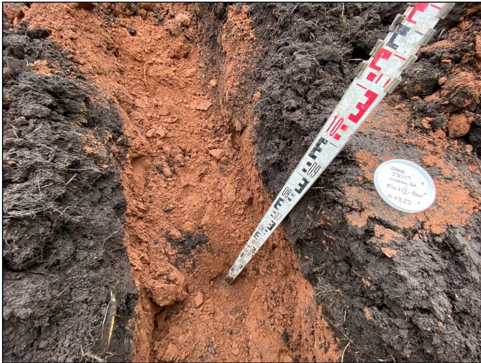
View of Plot 12 rear garden excavated to a depth of 0.95m exposing geotextile membrane at base.
