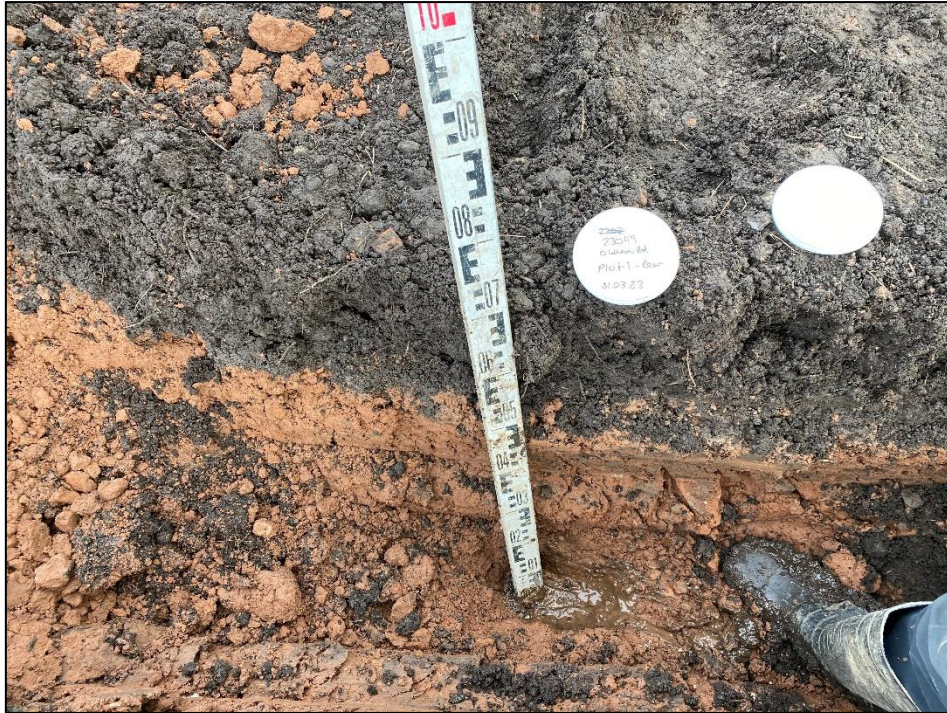
View of Plot 1 rear garden excavated to a depth of 0.75m exposing geotextile membrane at base.
