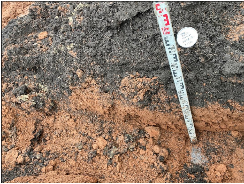
View of Plot 8 rear garden excavated to a depth of 0.80m exposing geotextile membrane at base.
