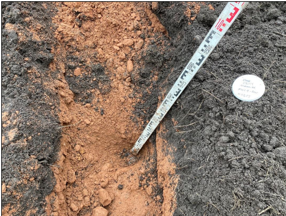
View of Plot 9 rear garden excavated to a depth of 0.80m exposing geotextile membrane at base.
