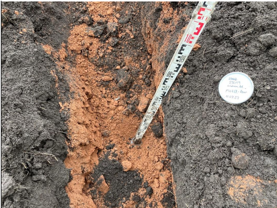
View of Plot 11 rear garden excavated to a depth of 0.90m exposing geotextile membrane at base.
