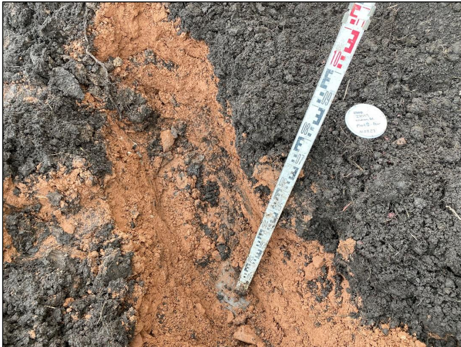
View of Plot 5 rear garden excavated to a depth of 0.80m exposing geotextile membrane at base.
