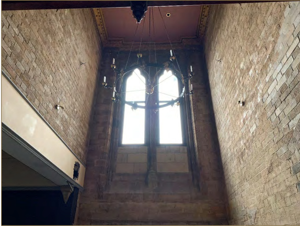
Photograph 27: View the former entrance hall window.
