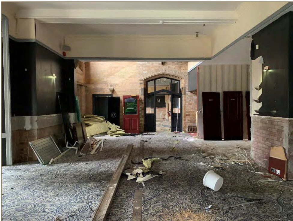
Photograph 30: View across internal dining room west.
