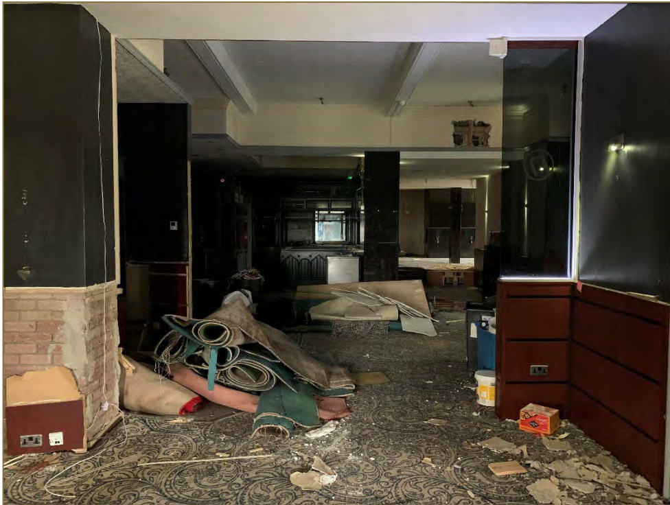
Photograph 39: View over bar area.
