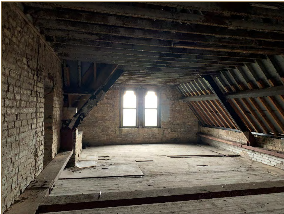
Photograph 44: View of second-floor attic.
