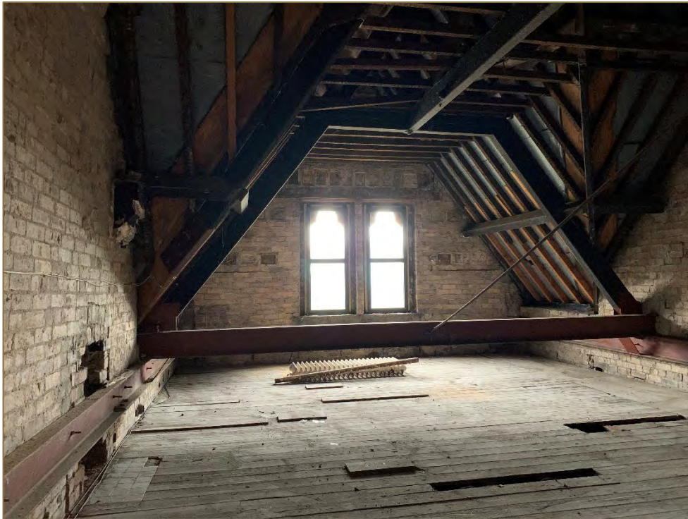
Photograph 43: View of second-floor attic.
