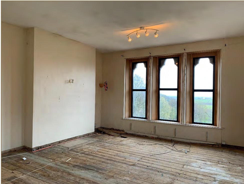
Photograph 41: View of first-floor room.
