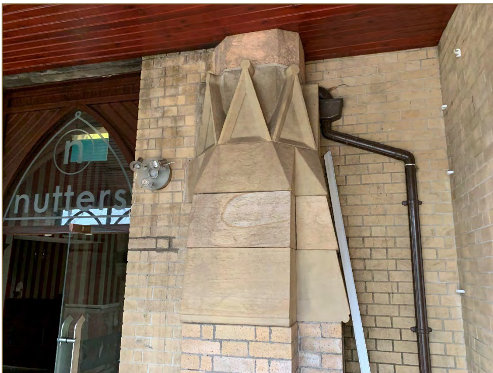
Photograph 36: View of possibly reclaimed capital on brick built column.
