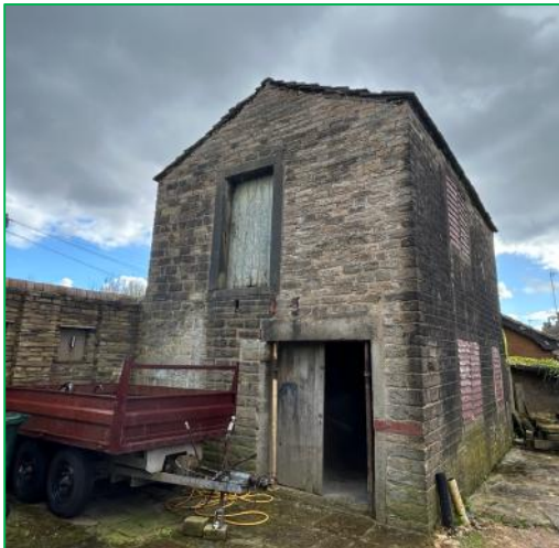
The northwest elevation of the building
