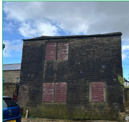
The southwest elevation of the building
