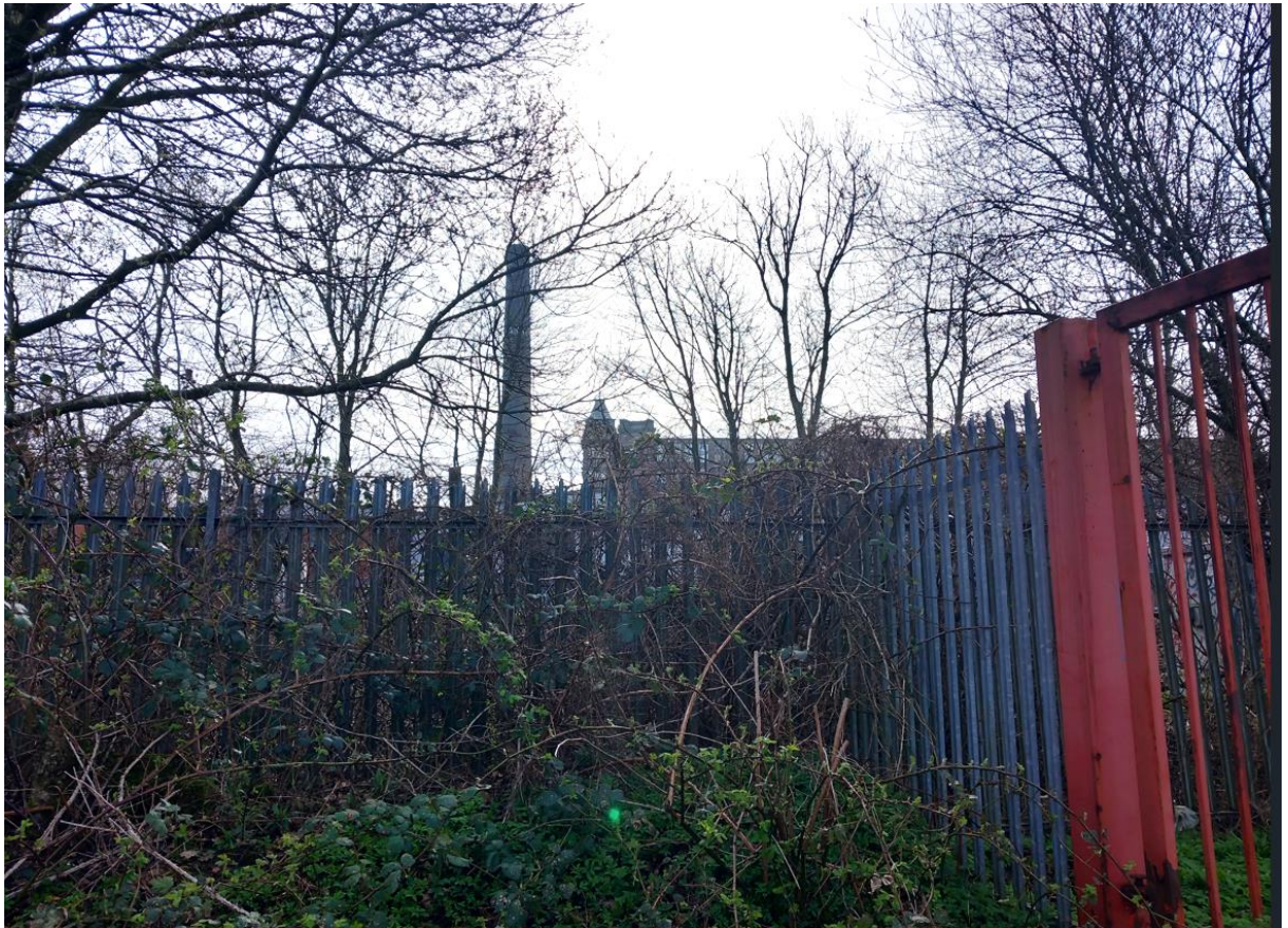
Plate 2: View of Arrow Vale Mill from Gipsy Lane. Photograph taken facing approximately SE.
