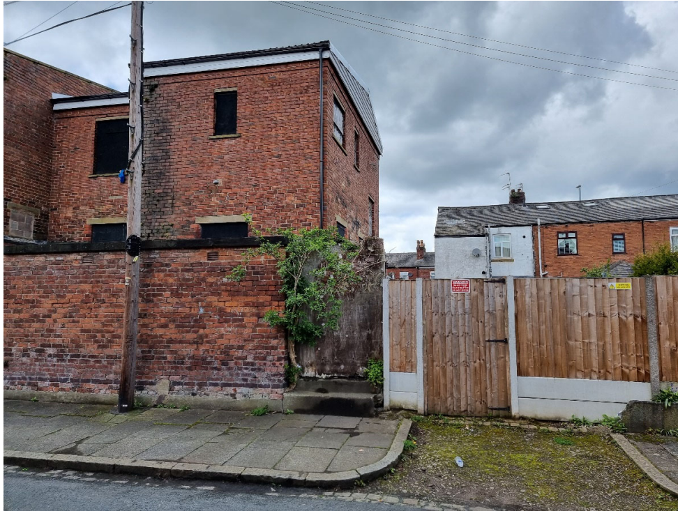
View from Pool Bank Street looking North
