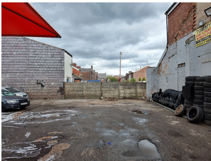
View from within the site looking East towards boundary to be infilled with screen wall
