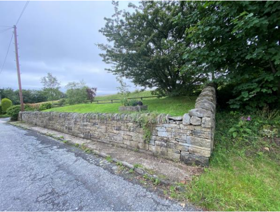
raised mound adjacent to Wildhouse Lane screens the site from passing traffic and offers some sense of enclosure
