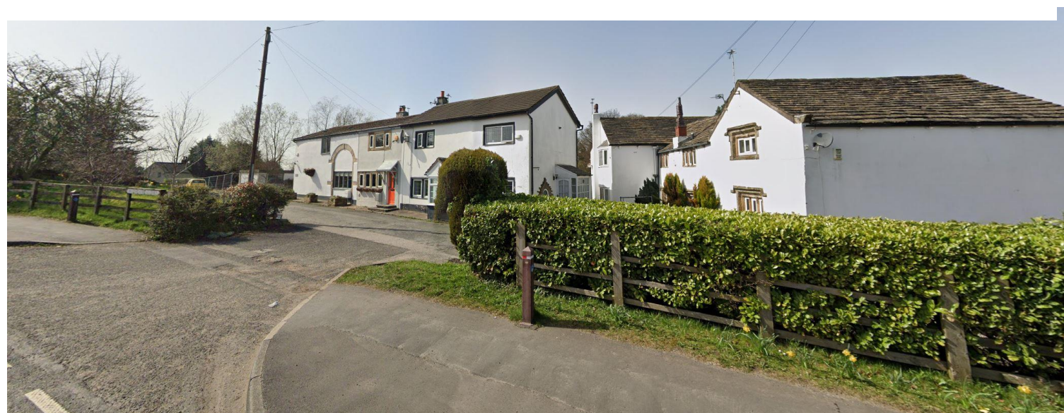
the front view is obscured by a mound and trees to Wildhouse Lane (the set-back and reduced ridge height will maintain this view)
