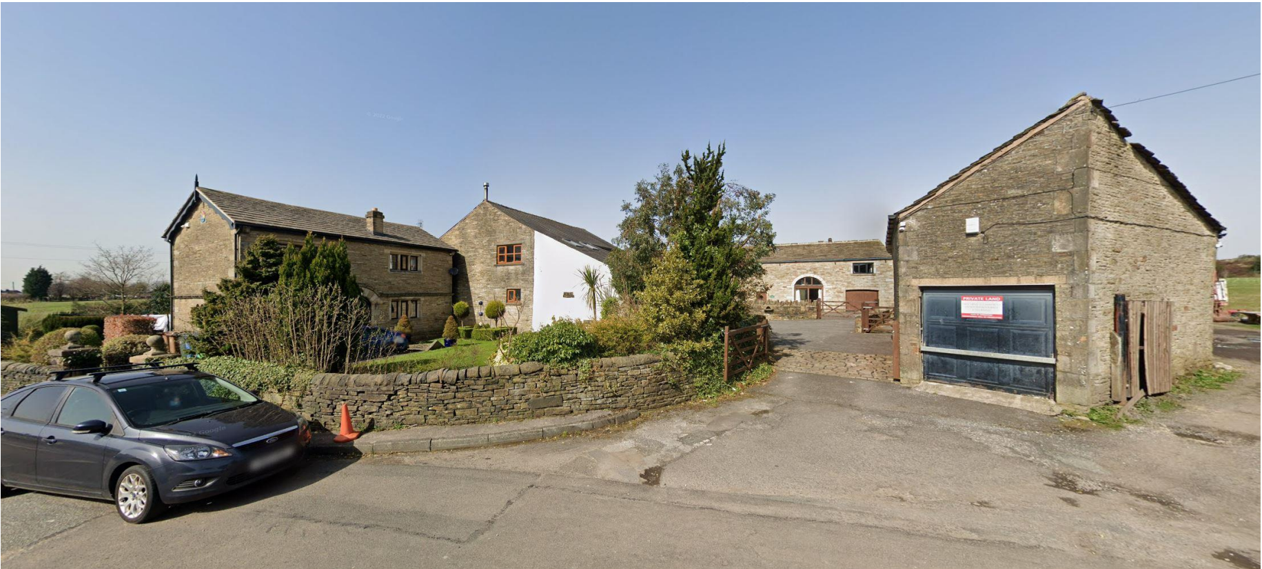
typical gable end frontages with a lean-to addition-Kiln Lane
