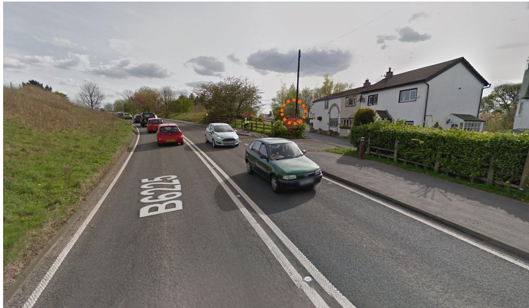
View of the site from the North of Wildhouse Lane
