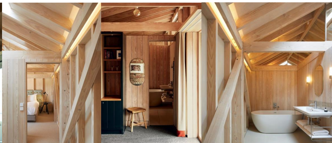
2. the roof structure is visible above the low-level partitions
