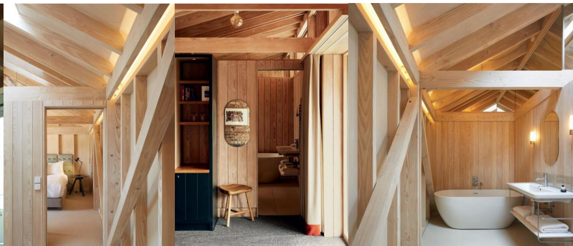
4. the roof structure is visible above the low-level partitions with a glass screen at the high level to the bedroom
