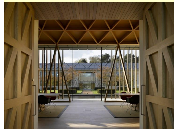
glulam roof structure
