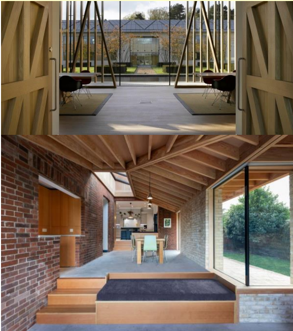
glulam roof structure and natural finishes express the structure internally as with traditional barns and cattle sheds
