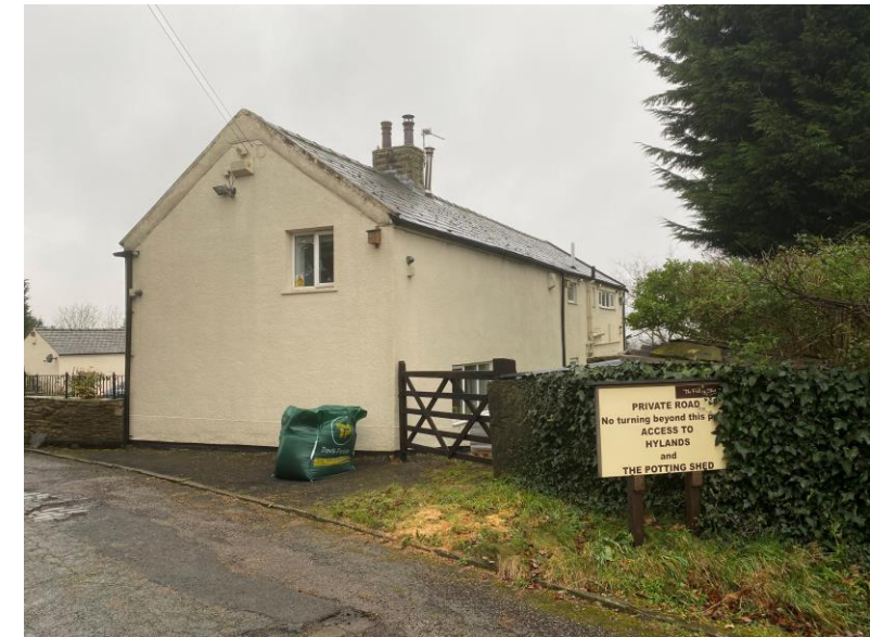
gable end frontage of the adjacent property
