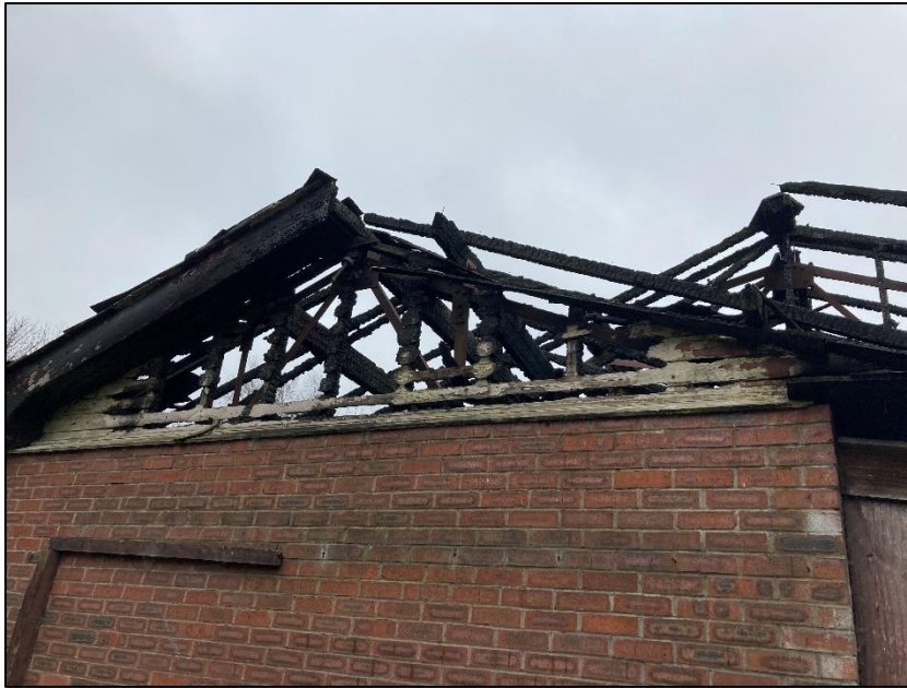
Photograph 13 showing the roof of the extension
