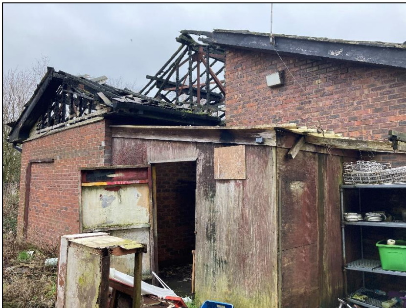
Photograph 14 showing the shed
