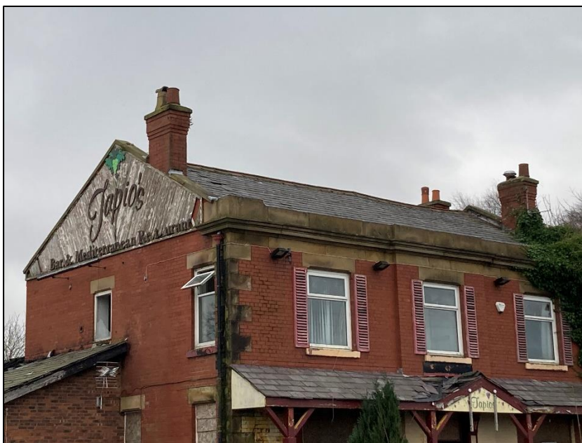
Photograph 12 showing the roof of the main building
