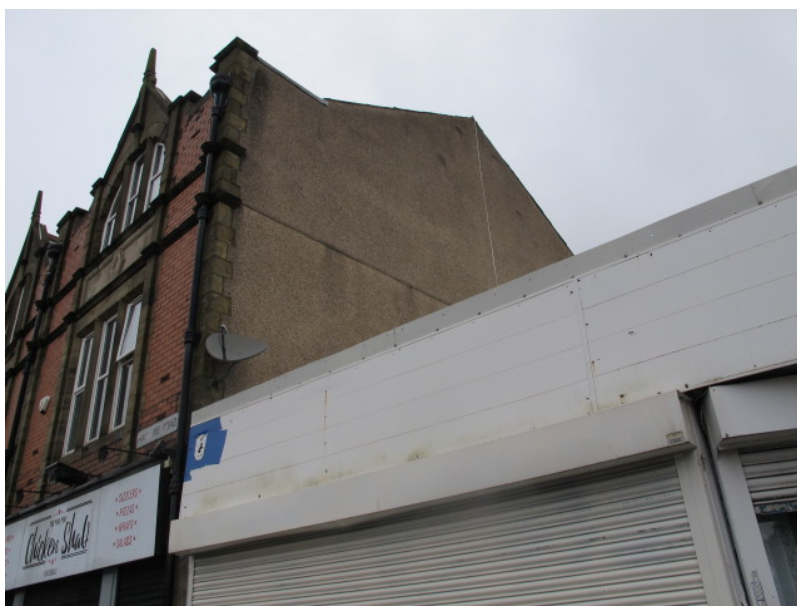
Photo 2 – Metal cladding to the roof and metal shutter
