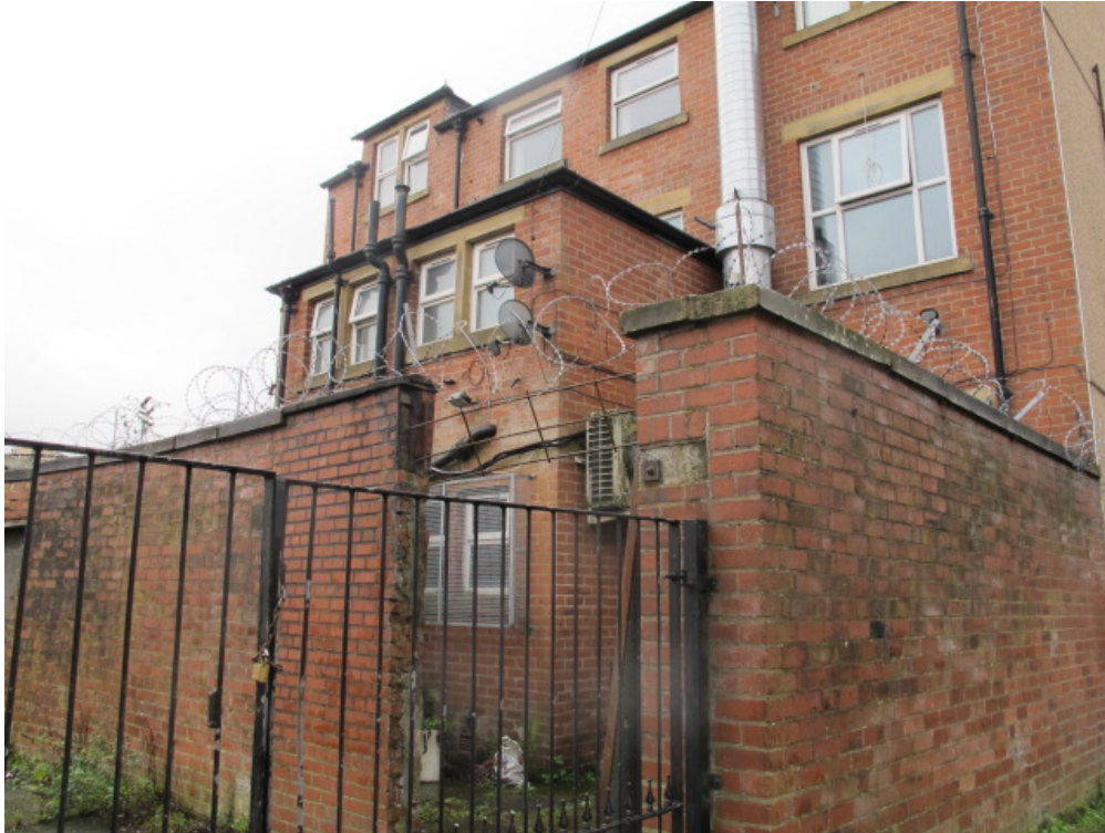
Photo 3 – Two-storey building proposed for demolition
