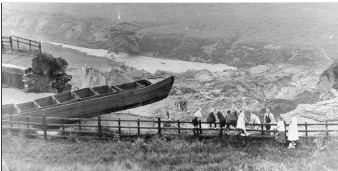
Figure 2-4: The 1936 canal breach from the North Bank
