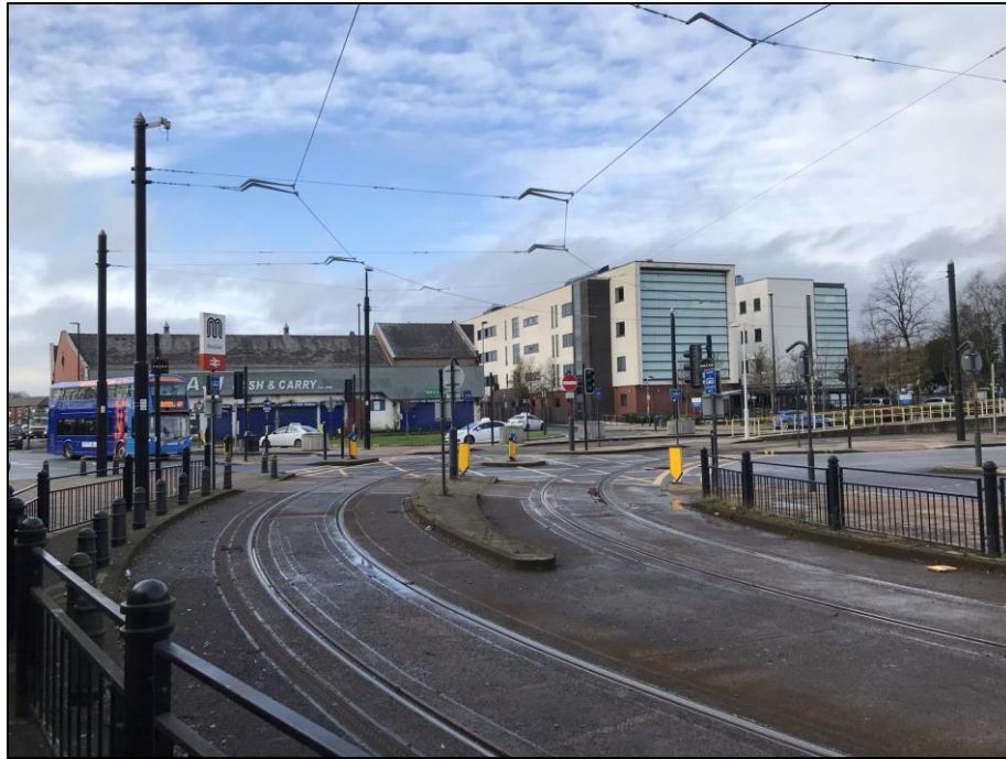
Fig 11 Typical view of urban infrastructure close to the station
