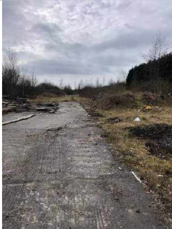
AREA OF HARD STANDING THROUGH CENTRE OF SITE – FACING SOUTH
