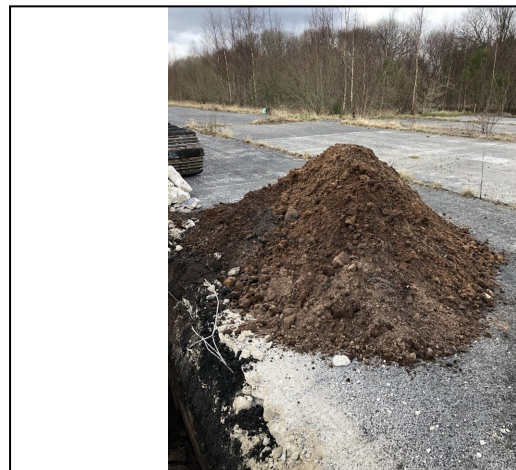
Trial Pit 109 Spoil
