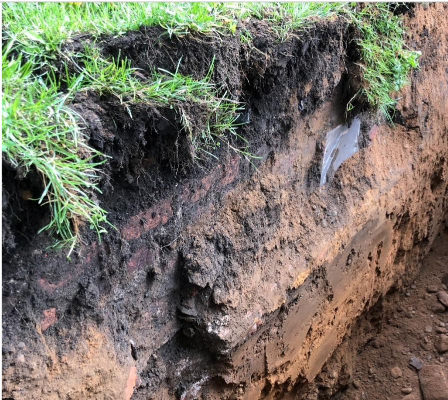
PLATE 4 HISTORIC FOUNDATIONS – TP101
