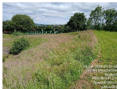
Embankment in the west of the site
