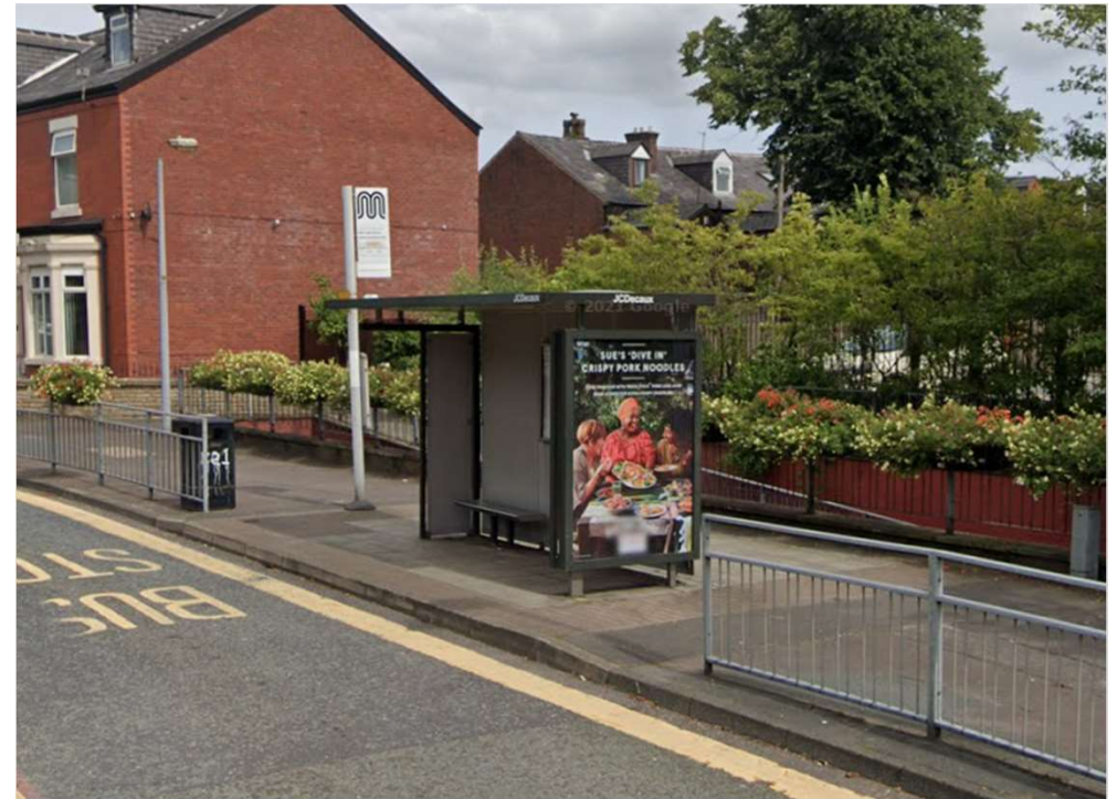
Southbound view of existing shelter
