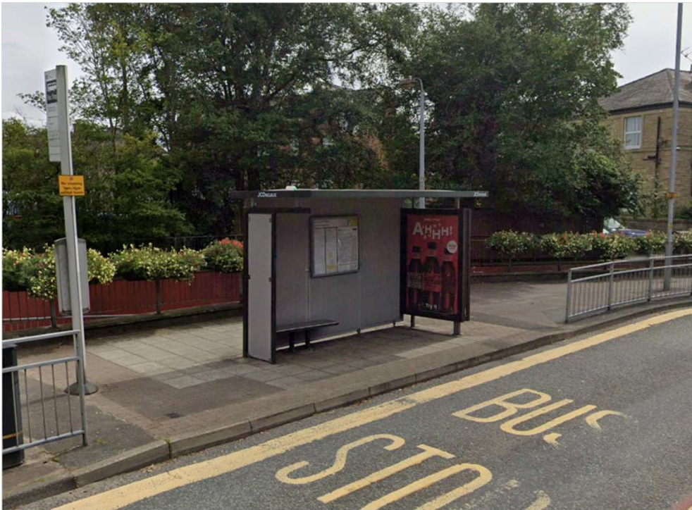
Northbound view of existing shelter
