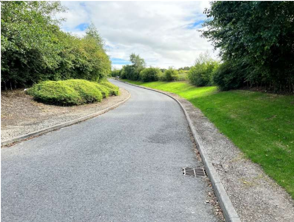
9. Looking back towards John Milne Roundabout
