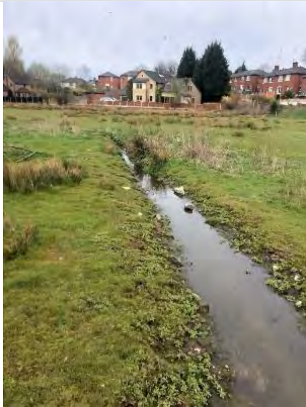
PLATE 6 DRAINAGE CHANNEL LEADING TO MANHOLES (SOUTHWEST)
