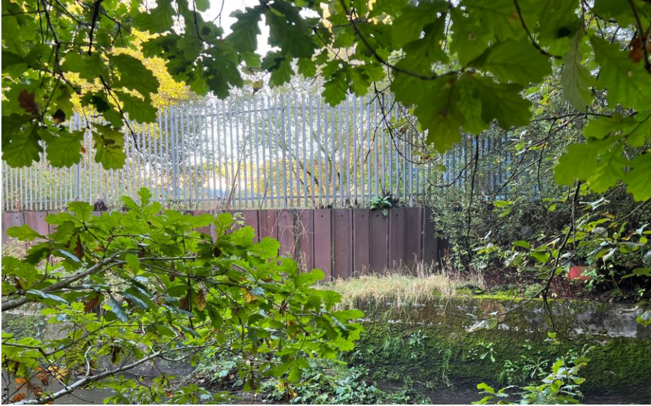
Site photographs of the boundary palisade fence.
