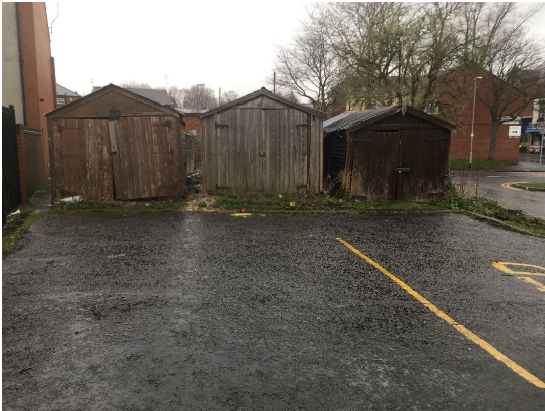
Photograph 3 – Block B garages.
