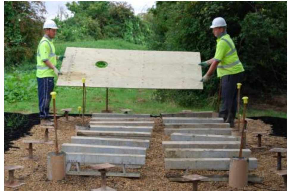
The Deck Support Units are covered with marine ply to provide the formwork for the concrete slab.
