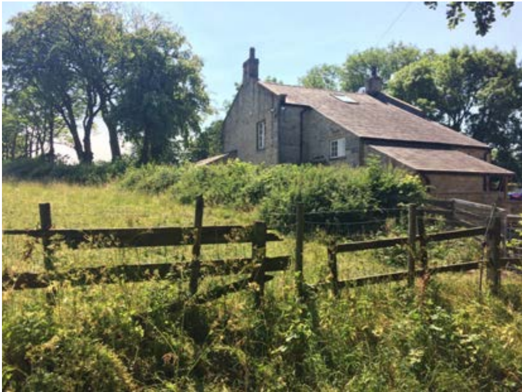
Plate 15: The rear view of the Grade II listed Clegg Hall House showing the rear outshut and servant's cottage.
