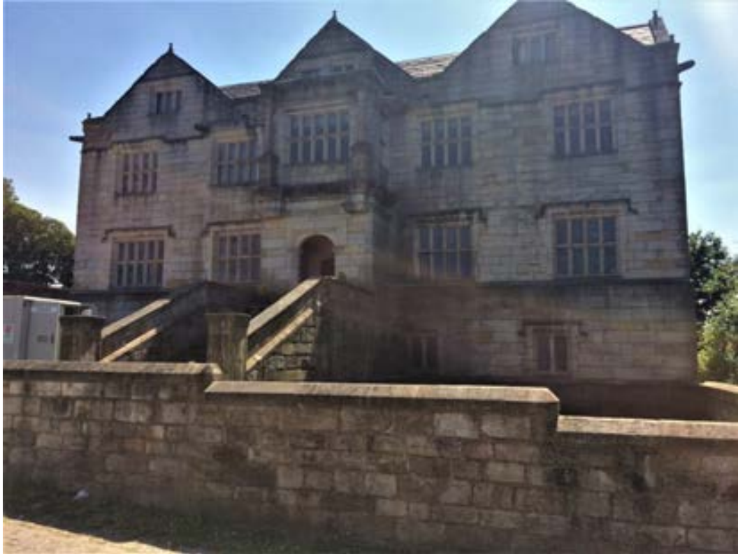
Plate 11: North-west facing façade of the Grade II* listed Clegg Hall.
