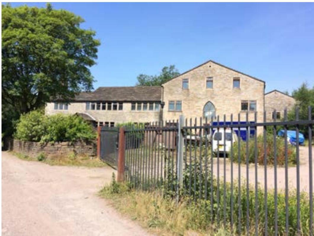
Plate 23: North-west facing view of the Grade II listed Lower Eafield Cottages, Barn and Stables from Clegg Hall Road.
