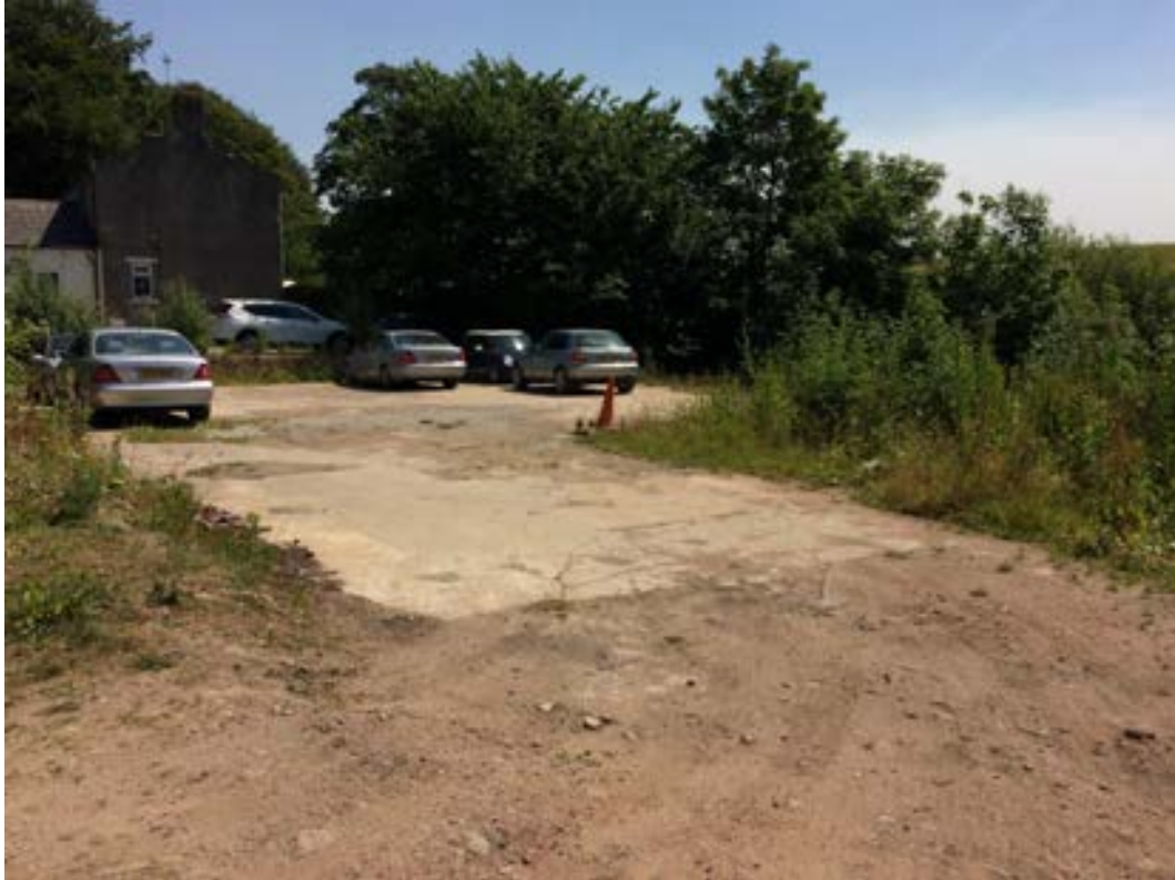
Plate 29: Hardstanding remains of the hand-loom weaving shed.
