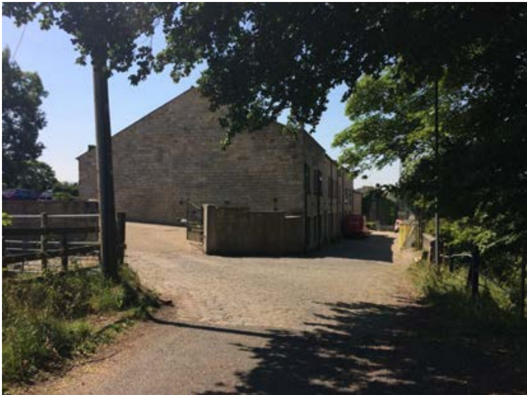
Plate 16: View south-west along Clegg Hall Road towards the gable end of the Grade II listed Clegg Mill Hall.
