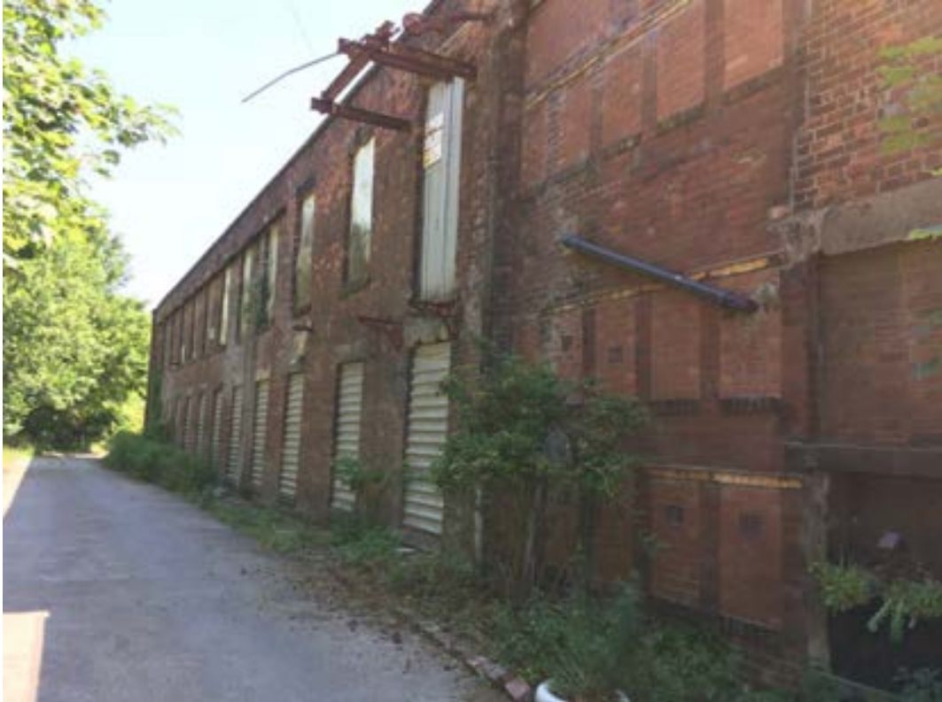
Plate 27: View along the north facing elevation of the mid-19th century mill range of the Dob Wheel Mill complex.
