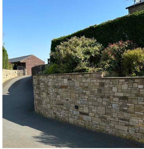
2. Existing Wall Retained
