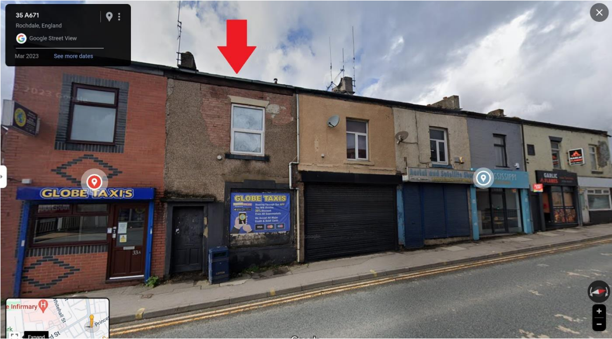
Red Arrow showing 35 Whitworth road with neighbouring buildings
