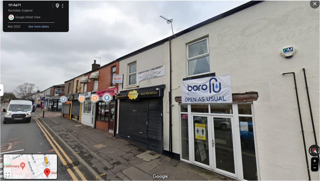
Buildings further up Whitworth road
