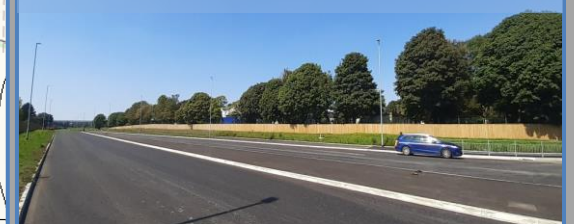
Looking north across the new link road towards the site
